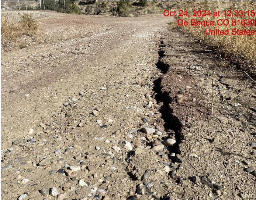
Insufficient Erosion Control on Lease Road – Photo #04495
