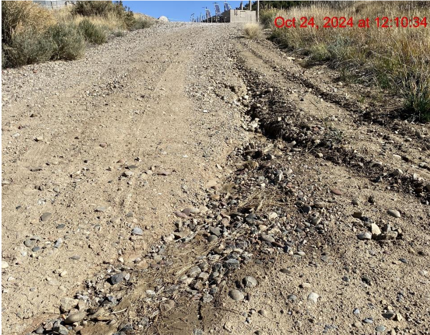
Insufficient Erosion Control – Photo #04473
