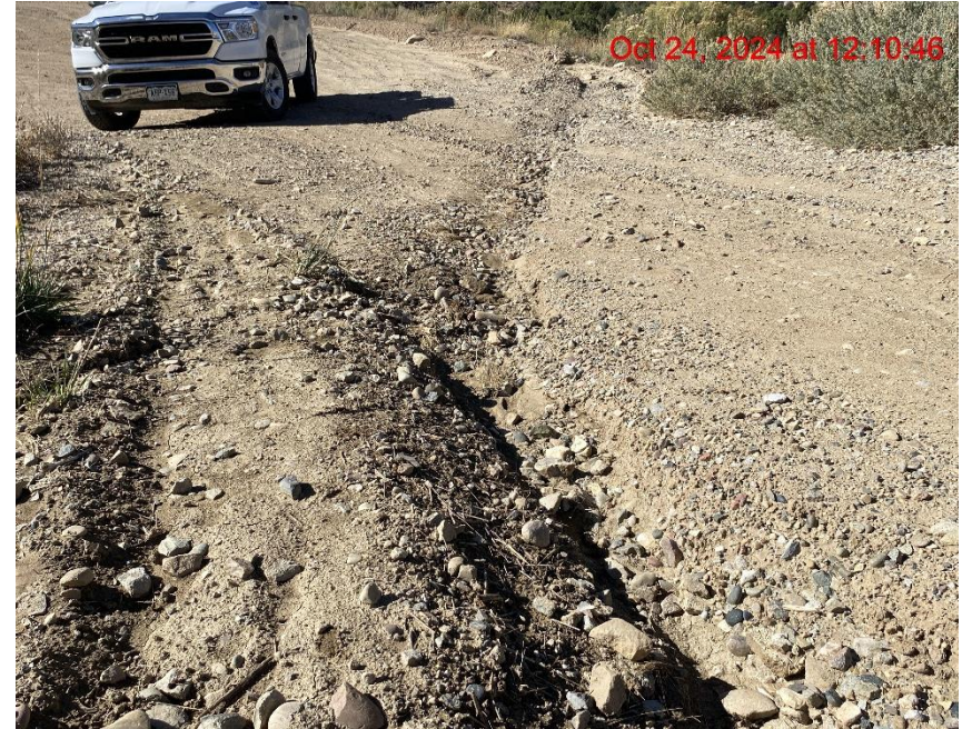
Insufficient Erosion Control – Photo #04474
