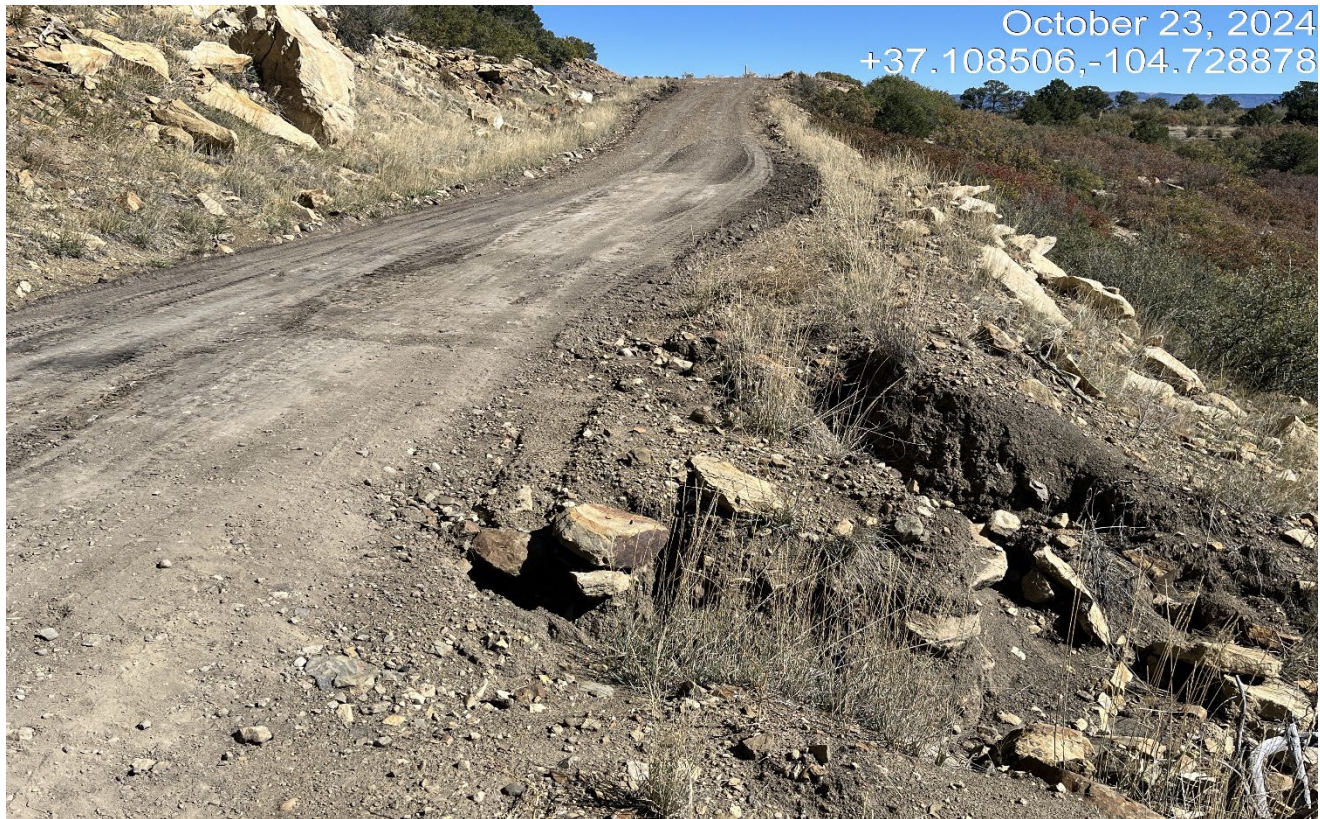
Photo 1. There is erosion along the access road northeast of the wellsite.
