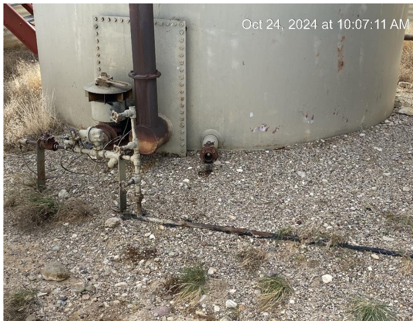
Open end tank valve. Stained soil.
