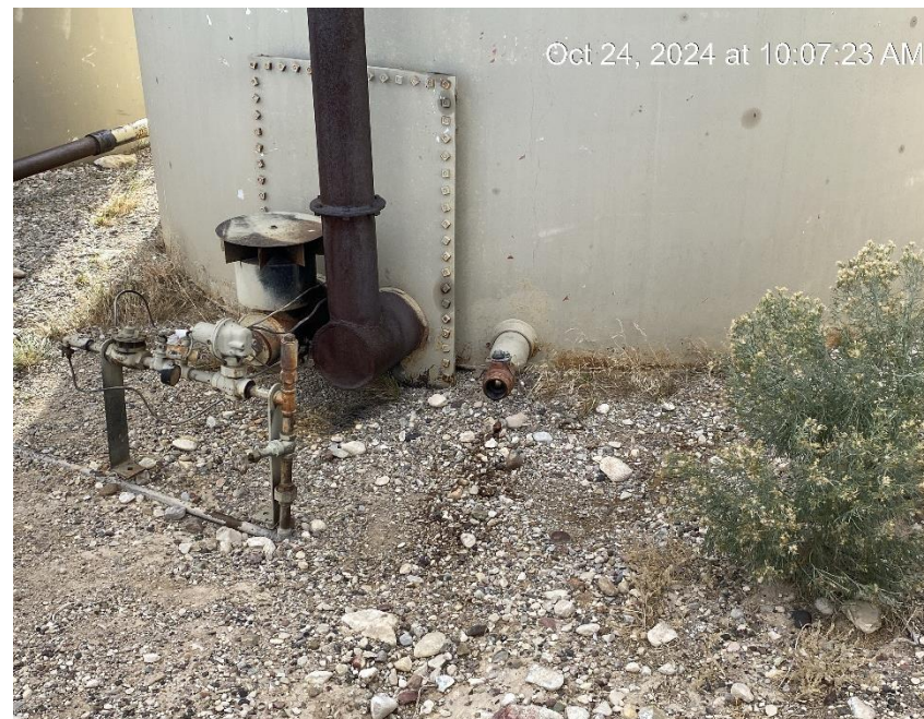
Open end tank valve. Stained soil.
