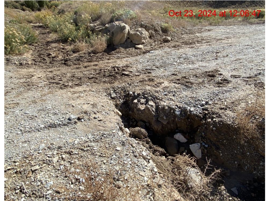
Insufficient Erosion Control/Degradation – Photo #04430
