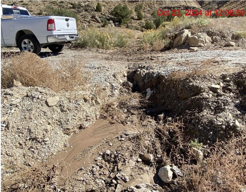
Insufficient Erosion Control/Degradation – Photo #04431
