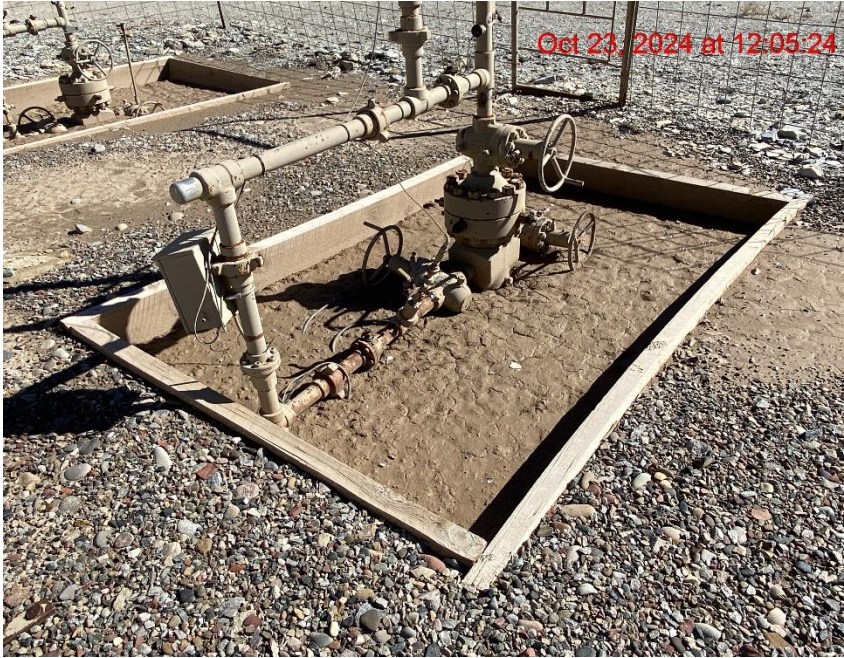
Open Wellhead Cellar/No Wildlife Egress – Photo #04428
