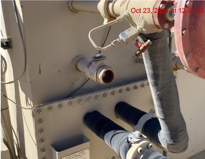
Open-Ended Line on Separator – Photo #04421
