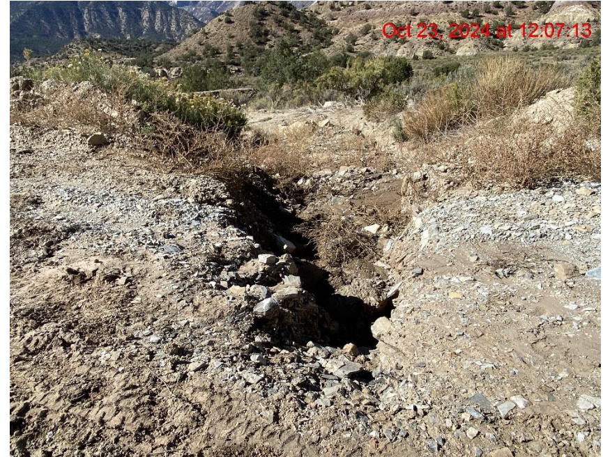
Insufficient Erosion Control/Degradation – Photo #04432
