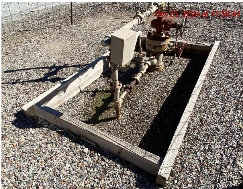
Open Wellhead Cellar/No Wildlife Egress – Photo #04418
