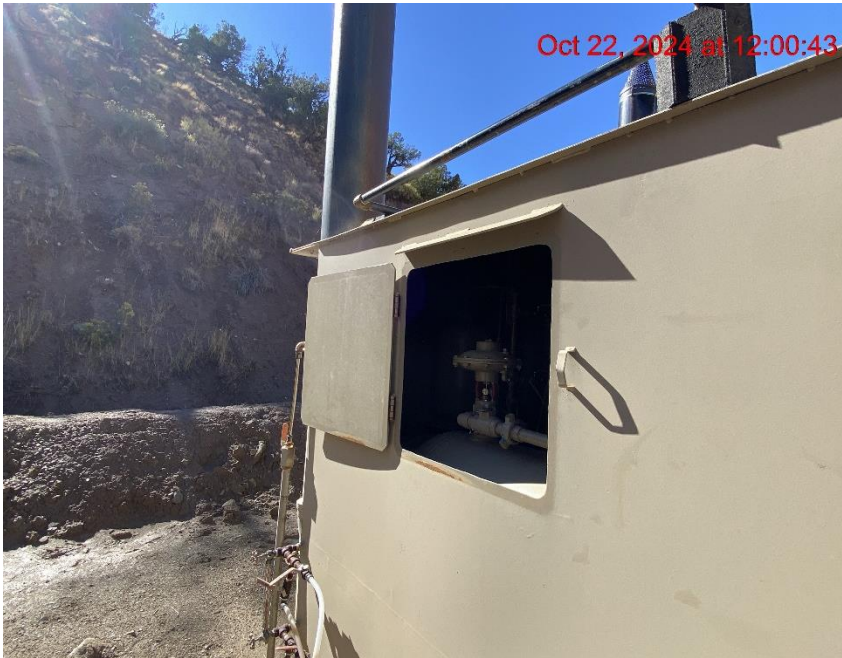
Unsecured Separator – Photo #04410
