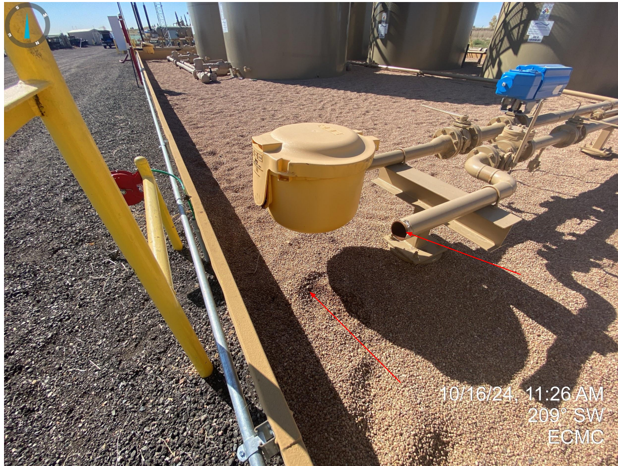
Photo 10. Stained soils and no observed bull plug at loadout line.
