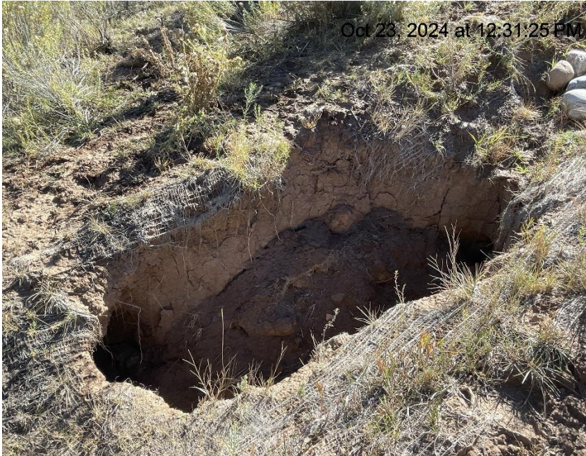
Photo # 6822 Subsidence in ditch/ditch needs maintenance
