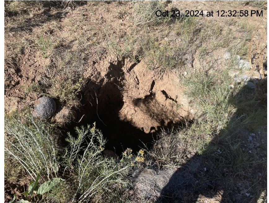
Photo # 6825 Subsidence in ditch/ditch needs maintenance
