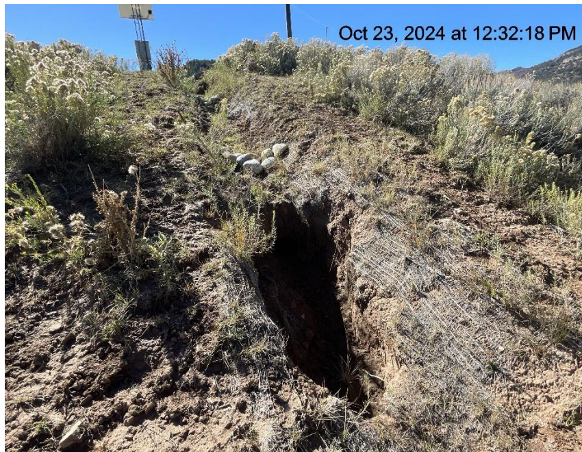
Photo # 6826 Subsidence in ditch/ditch needs maintenance
