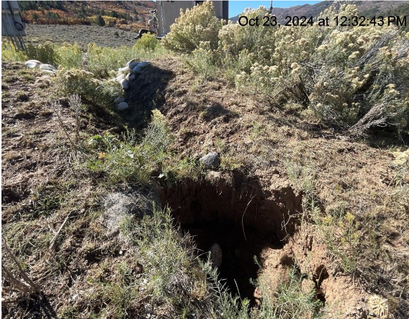
Photo # 6824 Subsidence in ditch/ditch needs maintenance
