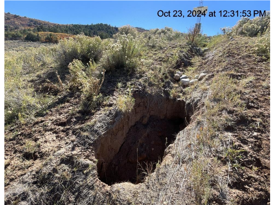
Photo # 6823 Subsidence in ditch/ditch needs maintenance
