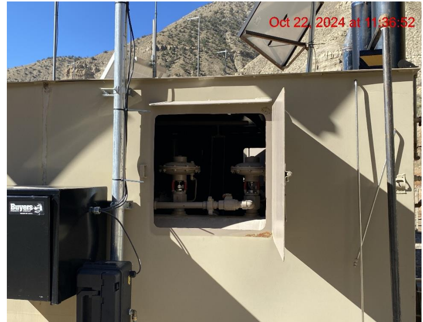
Unsecured Separator/Wildlife Entry Hazard – Photo #04372
