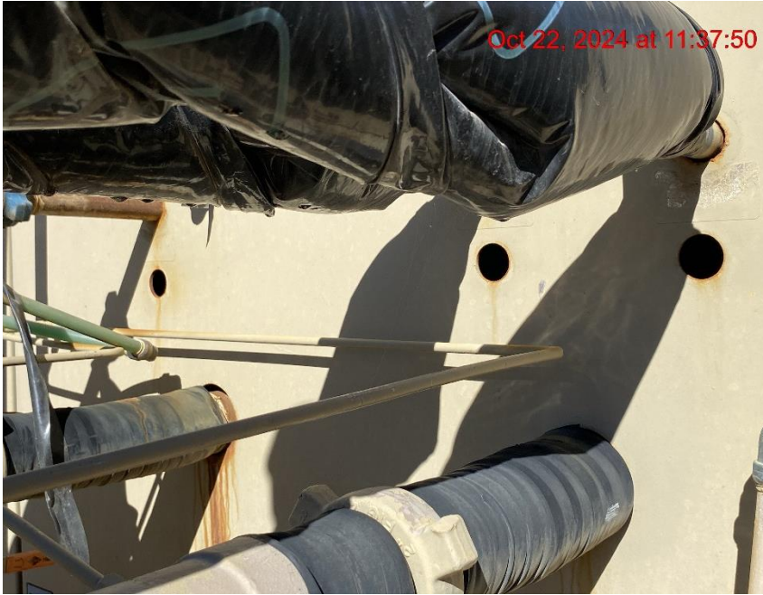
Separator/Wildlife Entry Hazard – Photo #04376
