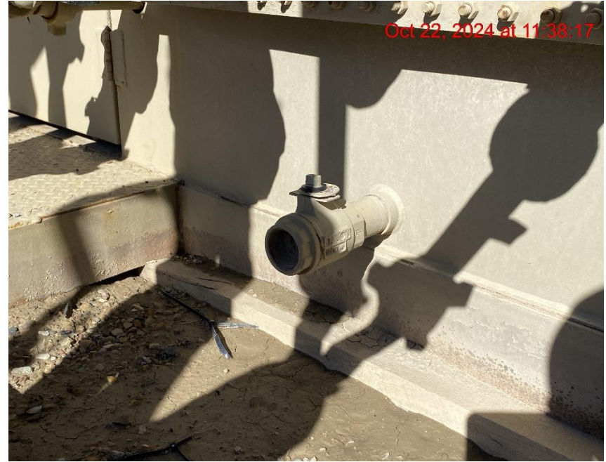
Open-Ended Line on Separator – Photo #04377
