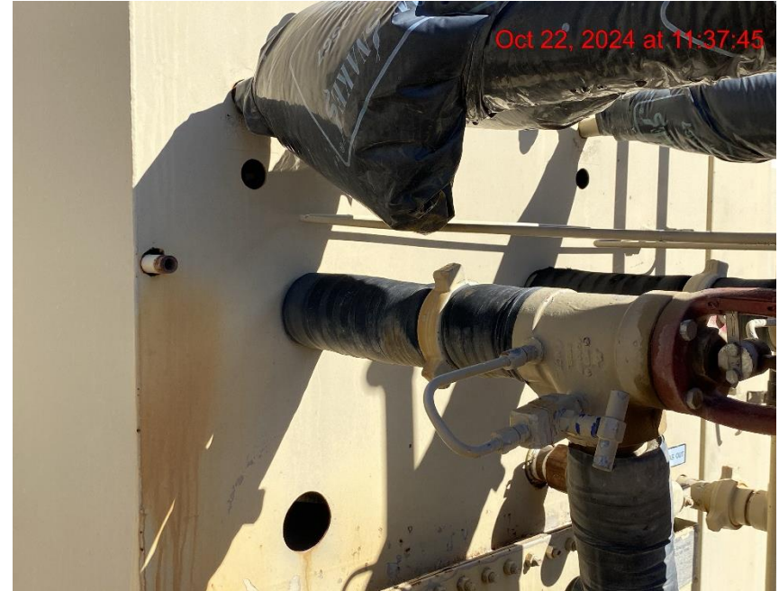
Unsecured Separator Separator/Wildlife Entry Hazard – Photo #04375
