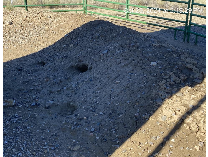
Burrows in tank berm
