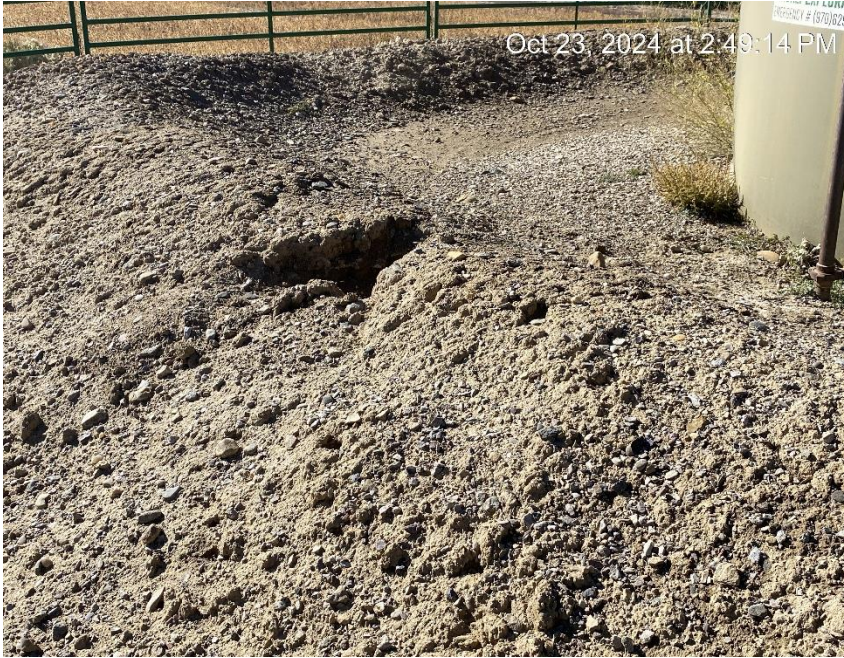
Burrow in tank berm
