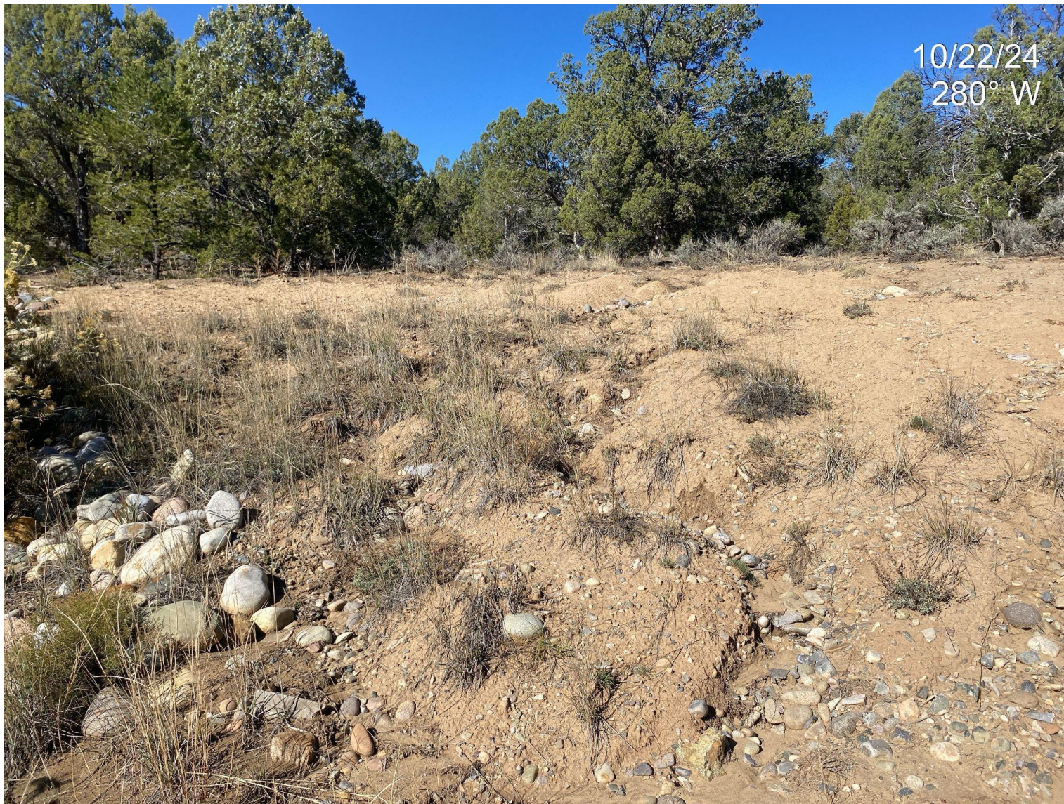
Photo 5. View of erosion forming along existing stormwater BMPs in the northwest corner of the disturbance. Additional stabilization/BMPs are needed in this area.
