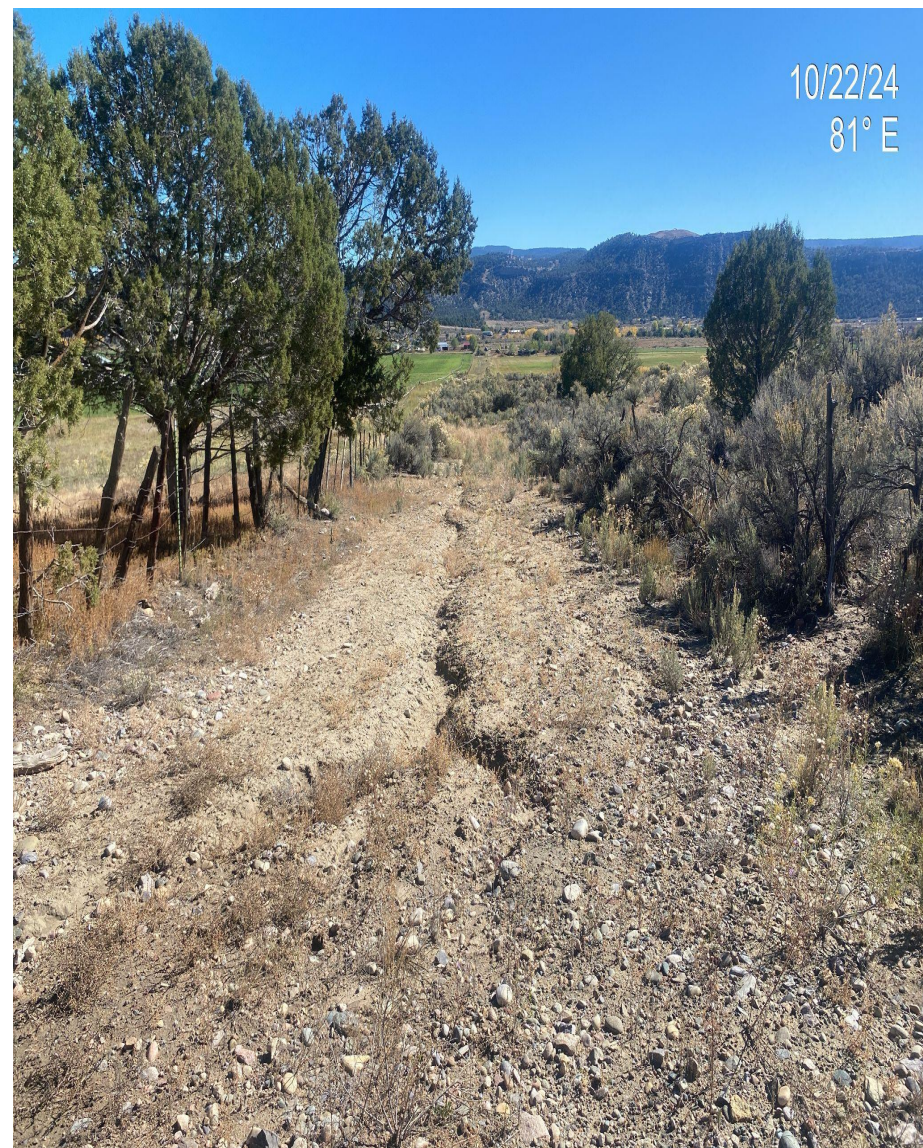
Photo 5. View of the access road that remains un reclaimed with bare soils, erosion issues and remnant rocks/gravel. Additional reclamation work along the access road is needed.
