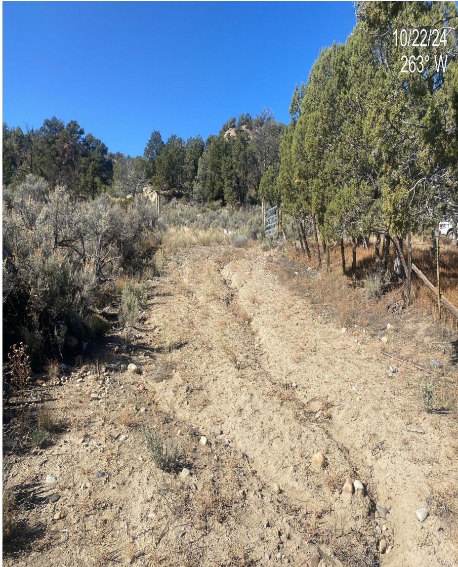
Photo 5. View of the access road that remains un reclaimed with bare soils, erosion issues and remnant rocks/gravel. Additional reclamation work along the access road is needed.
