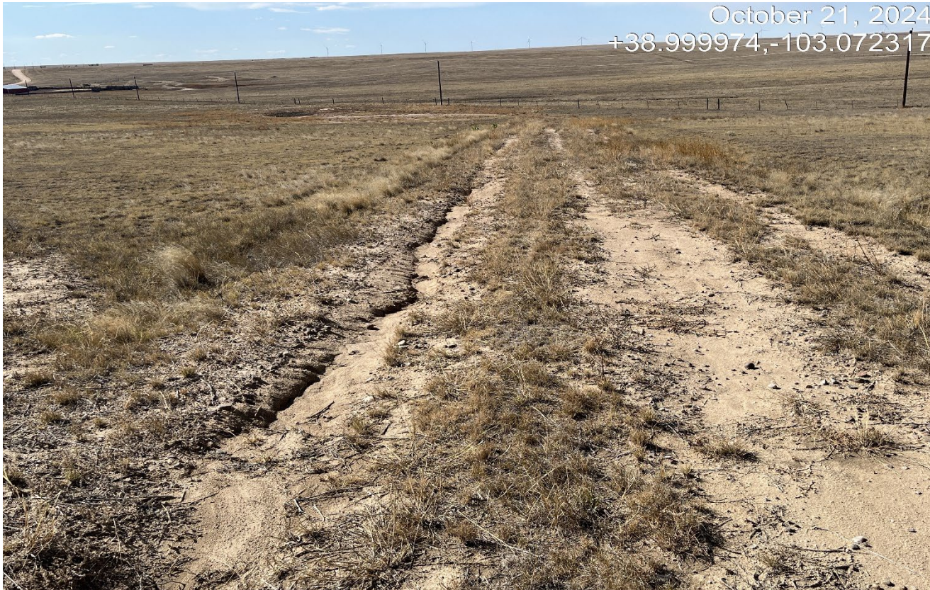
Photo 2. The access road is not recontoured and reclaimed. There is erosion occurring along this area of the road.
