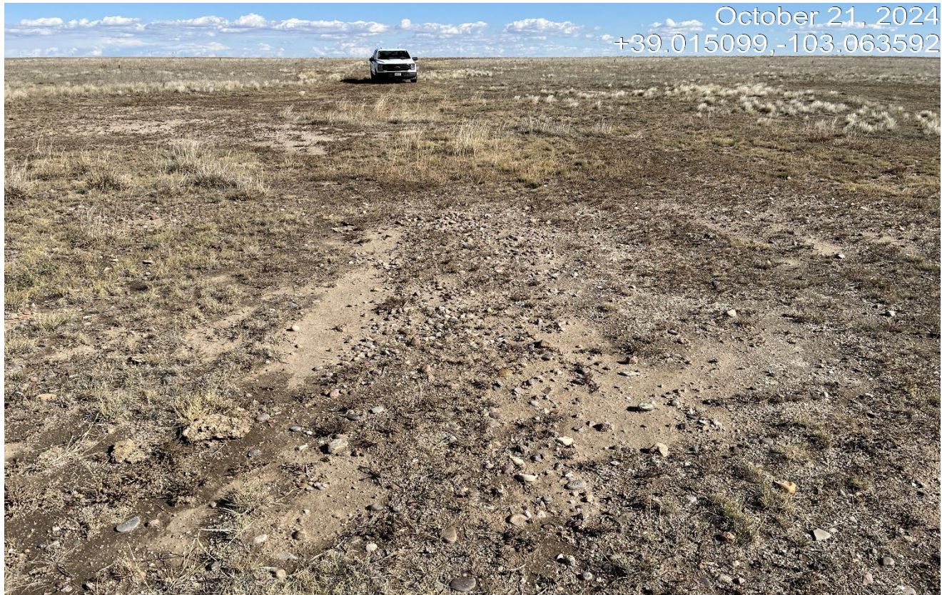
Photo 7. Facing east at the former wellsite. This area has compacted soils that need to be cross ripped.
