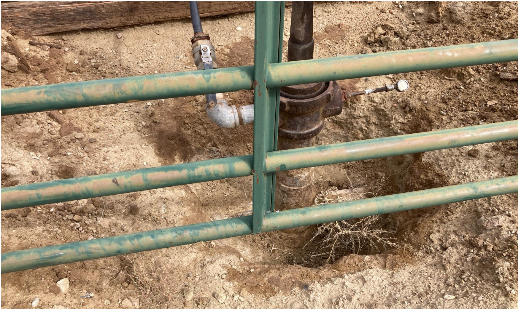
PHOTO 7: Bradenhead inaccessible or not visible( wellhead tree does not appear to include a Bradenhead in it original install). Install appropriate fittings to allow bradenhead visual inspection as per Rule 419.a.(1), (2). THIS IS THE SECOND NOTICE IMMEDIATE ACTION IS REQUIRED.
