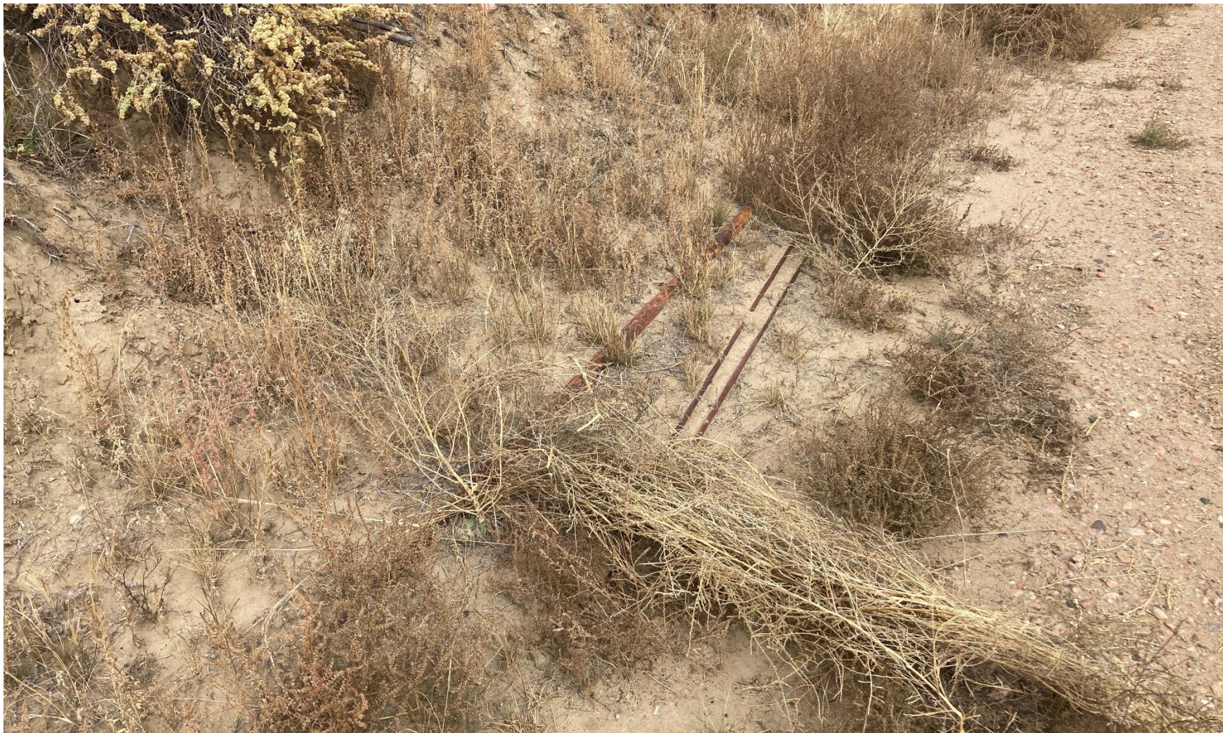
PHOTO 5: UNUSED EQUIPMENT (TUBING AND RODS ON WEST EDGE OF LOCATION), REMOVE UNUSED EQUIPMENT PER RULE 606. CA DATE 11/17/2024.
