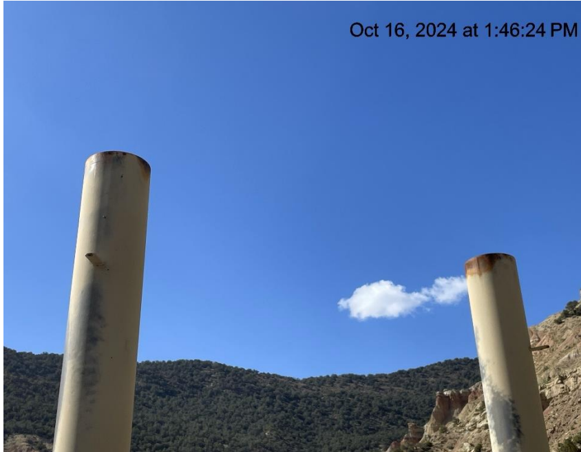
Photo # 6137 Burner exhaust stacks on separator units lack bird protection/wildlife hazard
