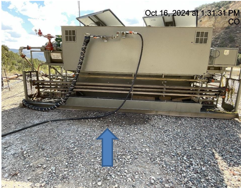
Photo # 6125 Staining near separator unit
