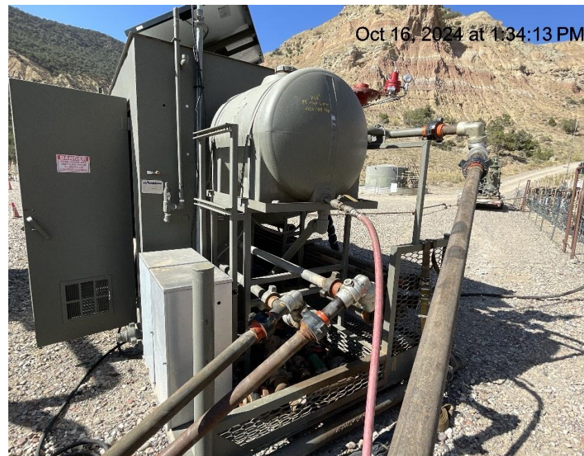
Photo # 6141 Chemical tank lacks BMP's
