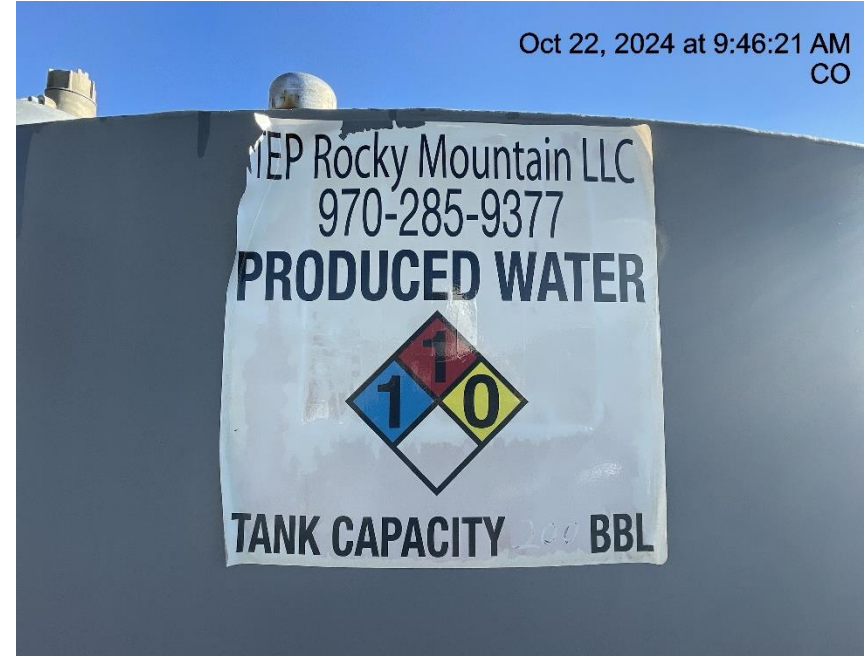
Photo # 6631 Capacity on tank label faded & illegible/tank label does not comply with CECMC rules
