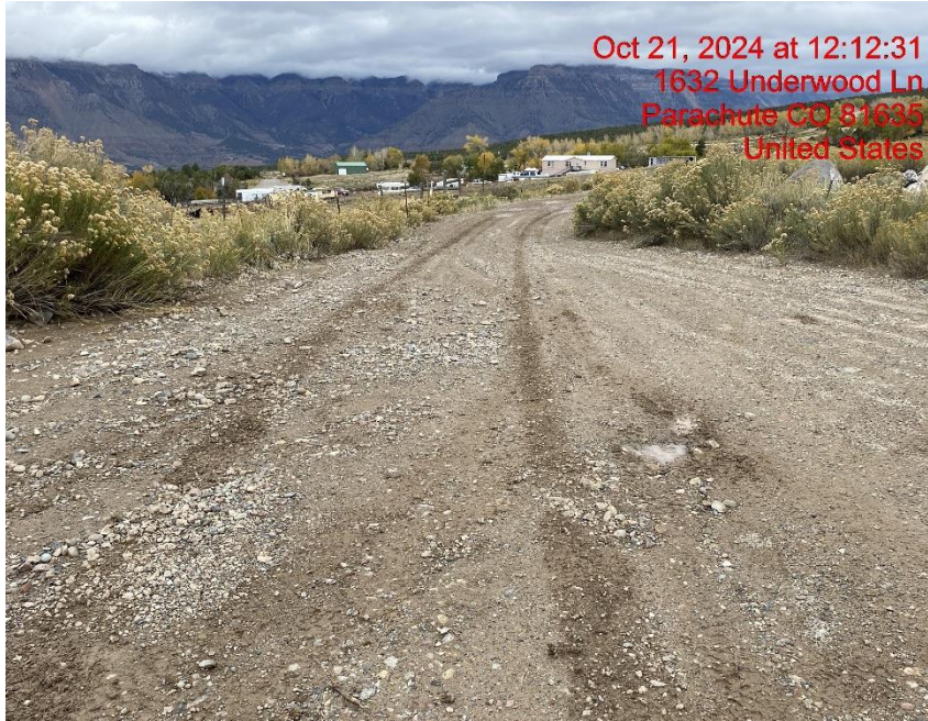
Insufficient Tracking BMPs – Photo #04324
