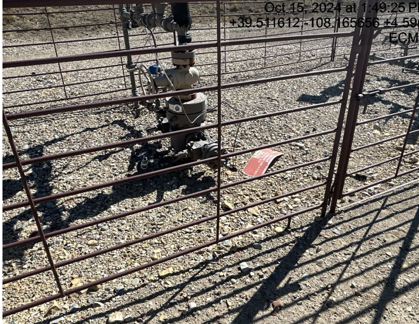
Well signage lacking information and on the ground
