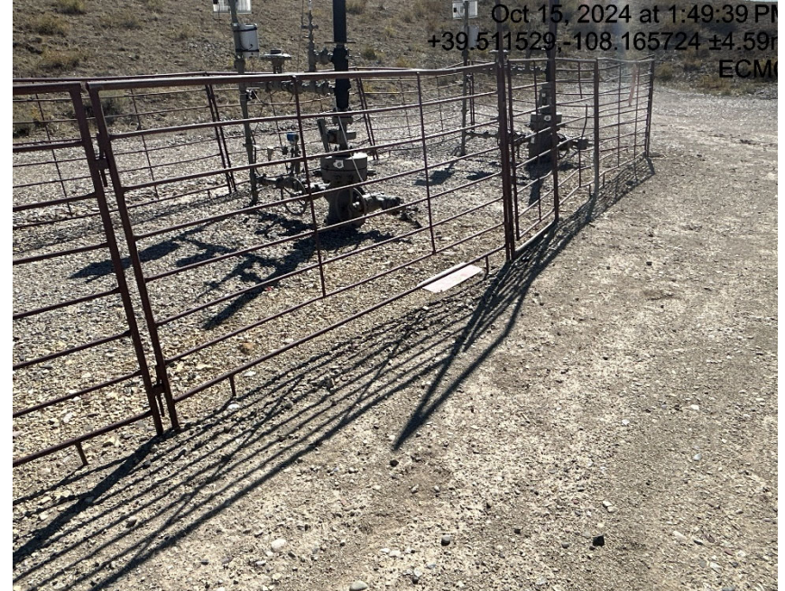
Well signage lacking information and on the ground
