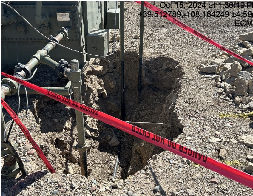
Open hole with minimal protection and open fencing
