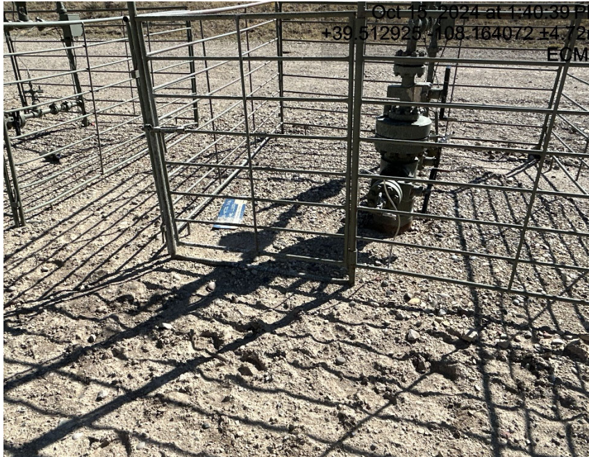
Well signage lacking information and laying on the ground
