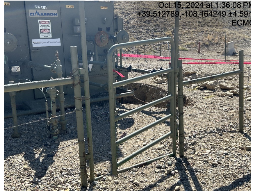
Open hole with minimal protection and open fencing
