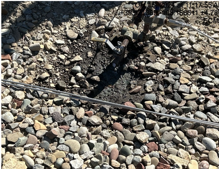
Leaking valve
