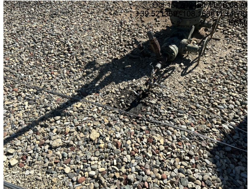
Leaking valve
