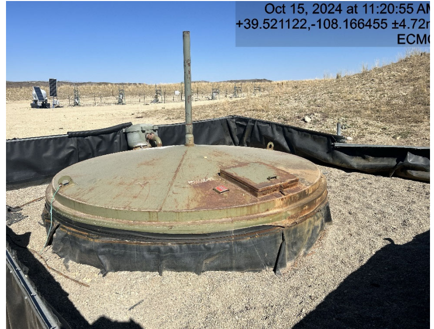
Condensate tank open to atmosphere
