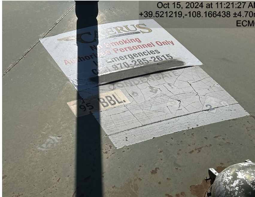
Condensate tank open to atmosphere
