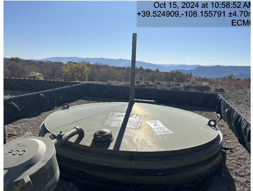
Condensate tank open to atmosphere
