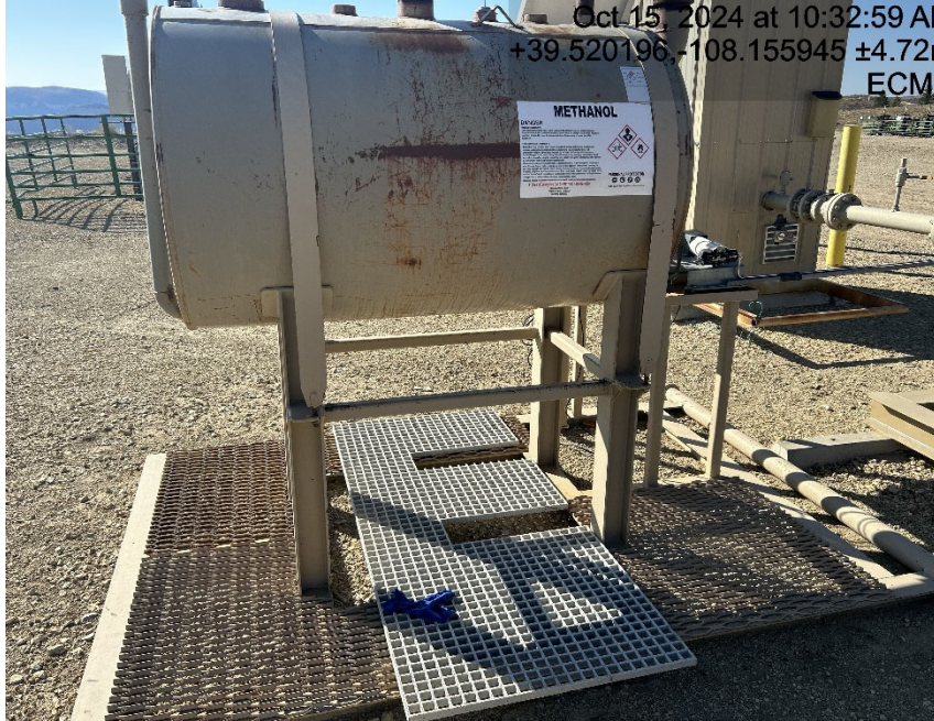
Tank lacking containment
