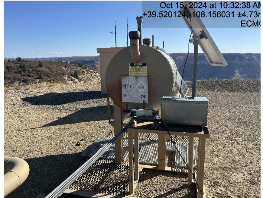
Tank lacking containment
