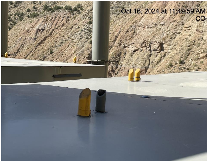
Photo # 5917 PRV vent line does not comply with CECMC pressure safety device rules
