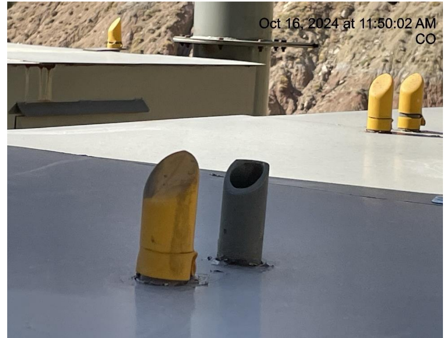
Photo # 5918 PRV vent line does not comply with CECMC pressure safety device rules
