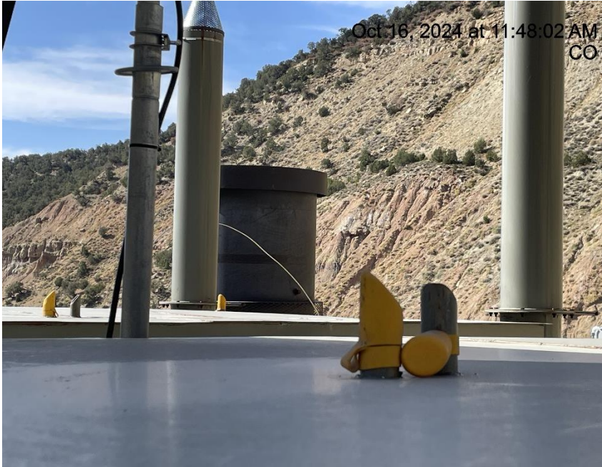
Photo # 5913 PRV vent line does not comply with CECMC pressure safety device rules
