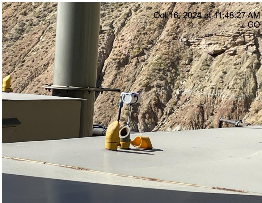
Photo # 5915 PRV vent line does not comply with CECMC pressure safety device rules
