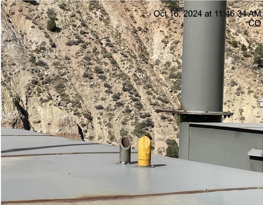
Photo # 5911 PRV vent line does not comply with CECMC pressure safety device rules
