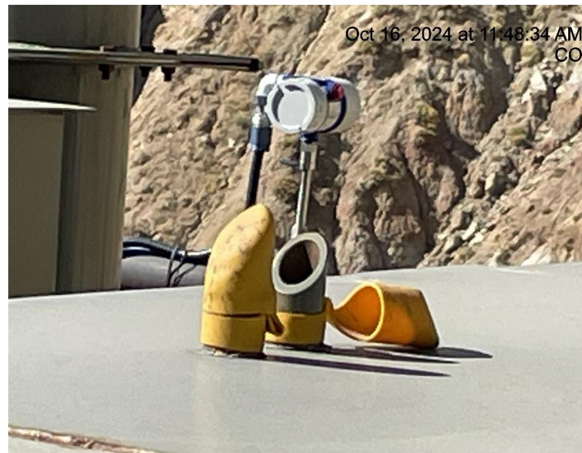
Photo # 5916 PRV vent line does not comply with CECMC pressure safety device rules
