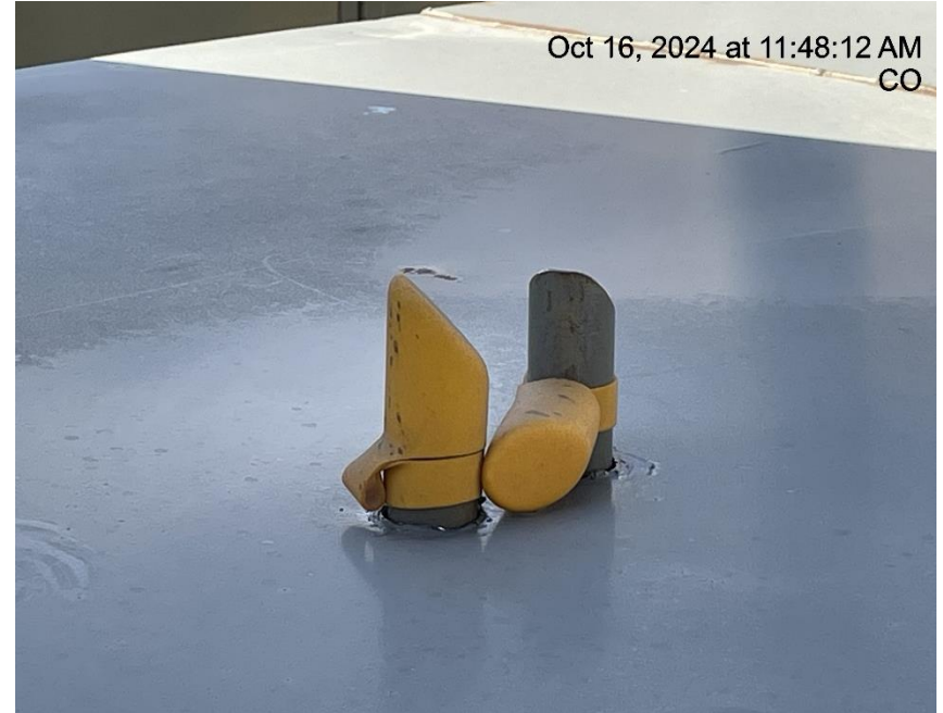
Photo # 5914 PRV vent line does not comply with CECMC pressure safety device rules
