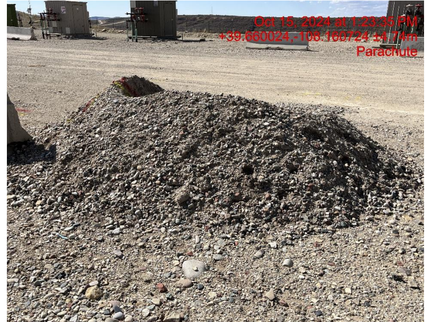
Photo # 7219 Stockpiled soils with no BMP's
