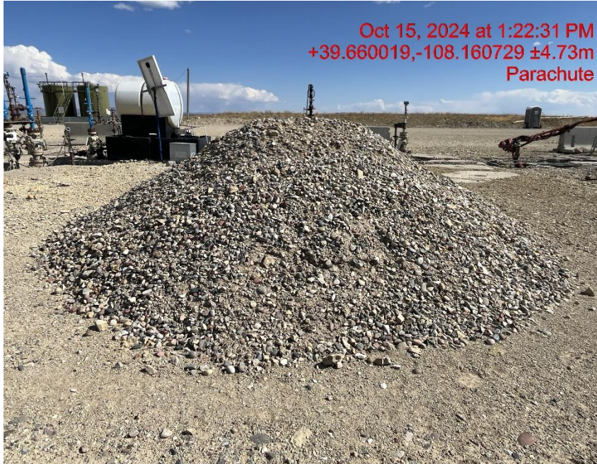
Photo # 7216 Stockpiled soils with no BMP's
