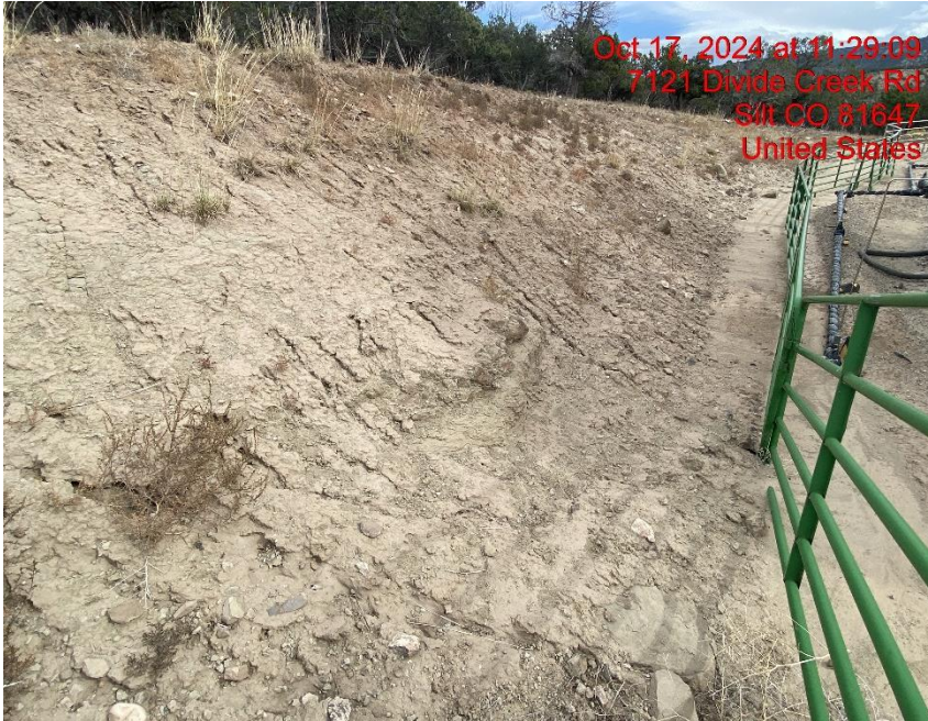
Insufficient Erosion Control – Photo #04276
