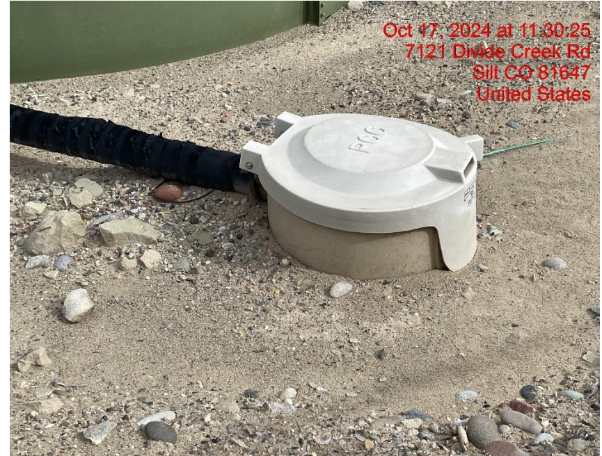
Sediment Encroaching Into Production Equipment/Degradation – Photo #04280
