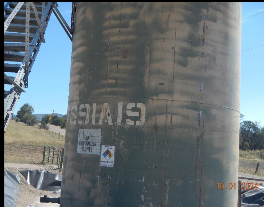
Tank labeling 10/1/24 with zero for flammability in NFPA diamond
