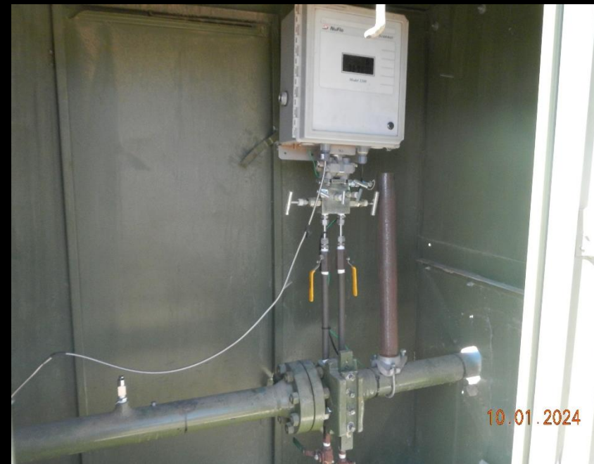
No calibration record displayed for 2A well 10/1/24
