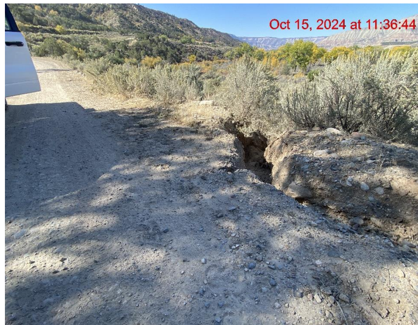
Insufficient Erosion Control – Photo #04234
