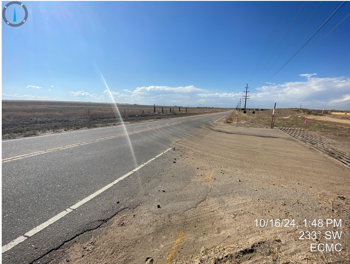
Photo 3. Sediment is beginning to collect at the location entrance and transferring onto the adjacent roadway. Additional BMPs/maintenance is required.
