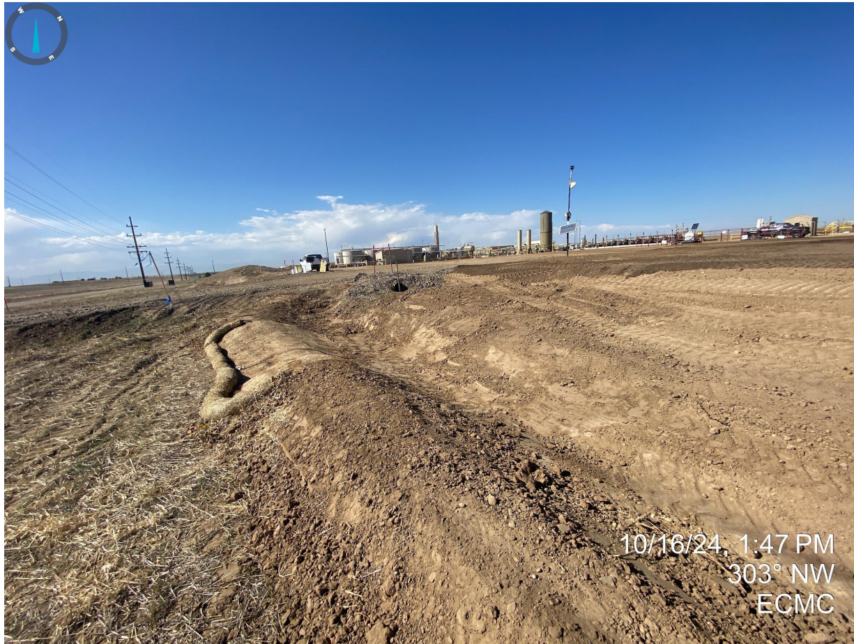
Photo 11. Sediment trap located near the southern portion of the drilling pad, east of entrance.
