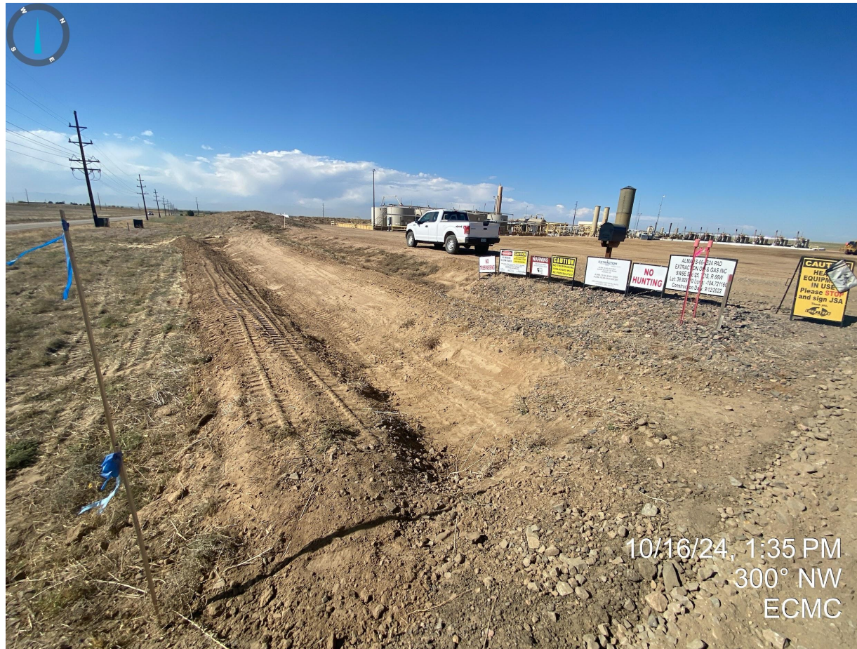
Photo 4. Sediment trap located near the southern portion of the drilling pad, west of entrance.
