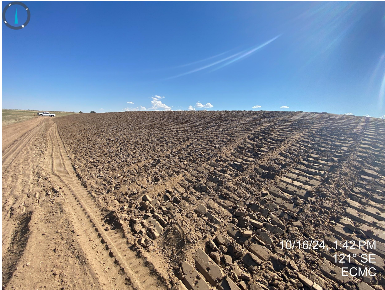
Photo 7. Appears that topsoil has been salvaged from the eastern interim areas as part of a drilling pad expansion. The topsoil stockpile appears to have been equipment tracked for short term stabilization.
