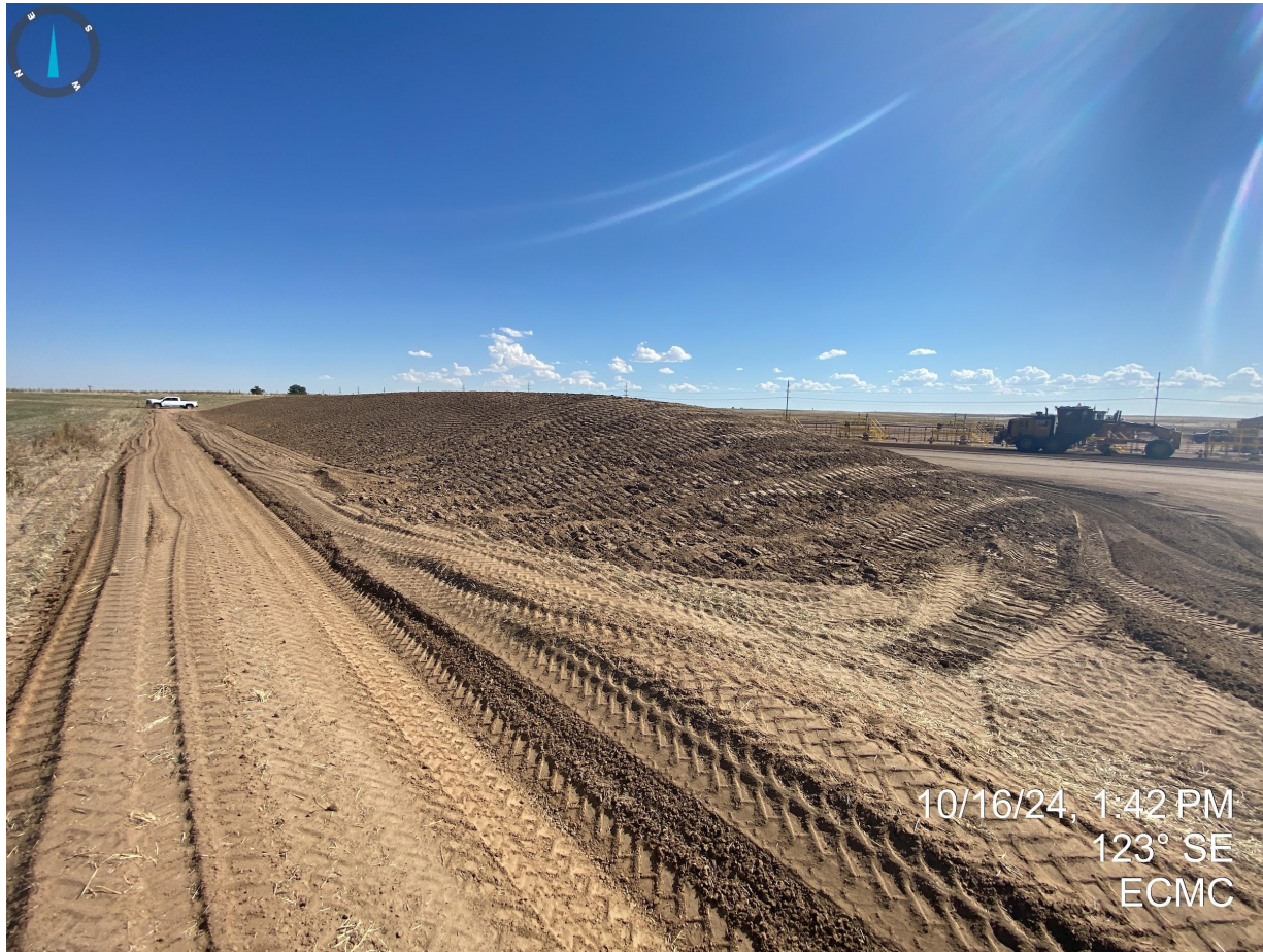
Photo 6. Ditch and berm has been constructed around the perimeter of the location.
