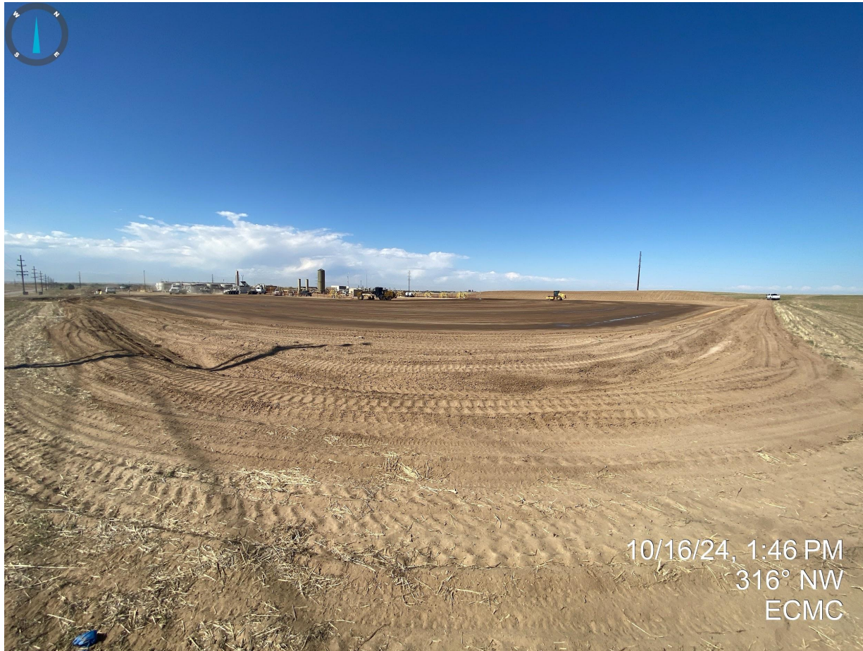
Photo 10. Taken from the southeast corner of the location. Photo illustrates perimeter ditch and berm constructed.
