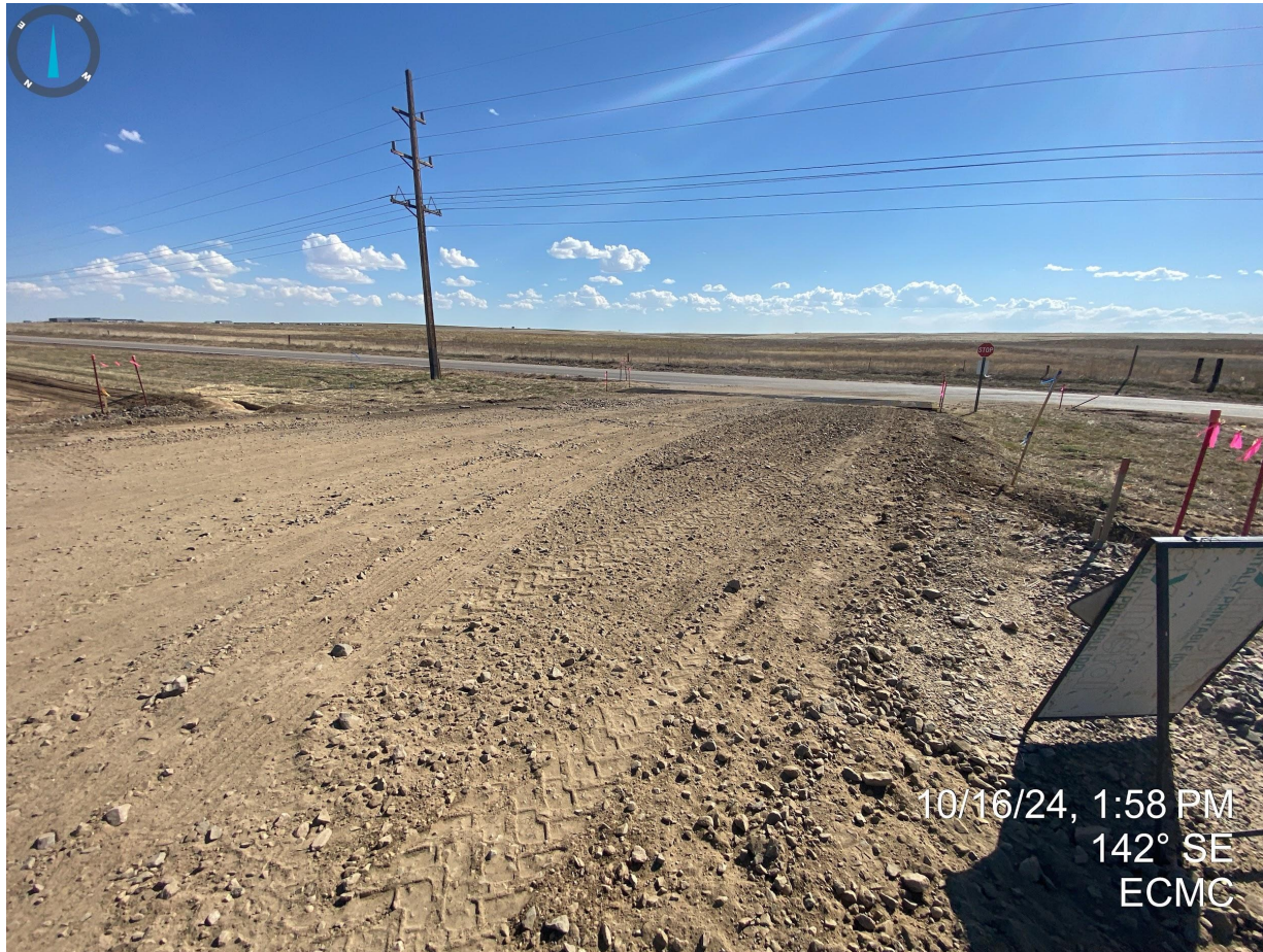
Photo 2. Vehicle track out pad at the location entrance requires maintenance.
