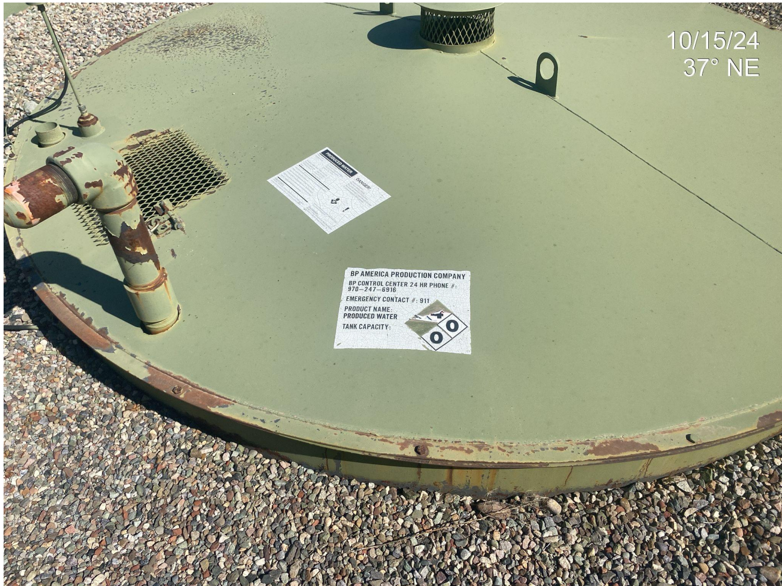
Photo 4. View of produced water tank label that is deteriorating and no longer displaying tank capacity.
