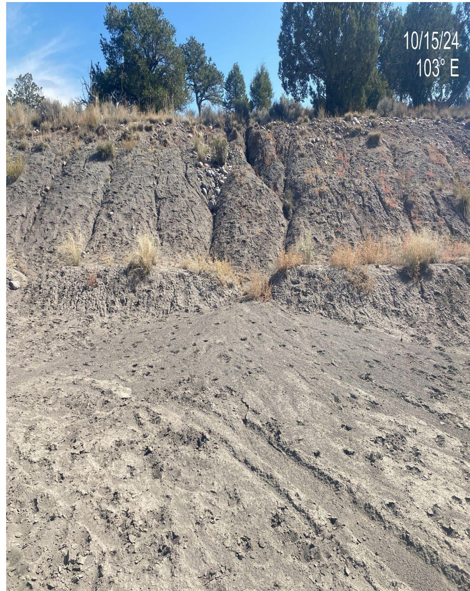
Photo 3. View of the eastern interim reclamation/cut slope. Area is lacking vegetation with evidence of gully erosion and sediment transport/deposition on the active pad.
