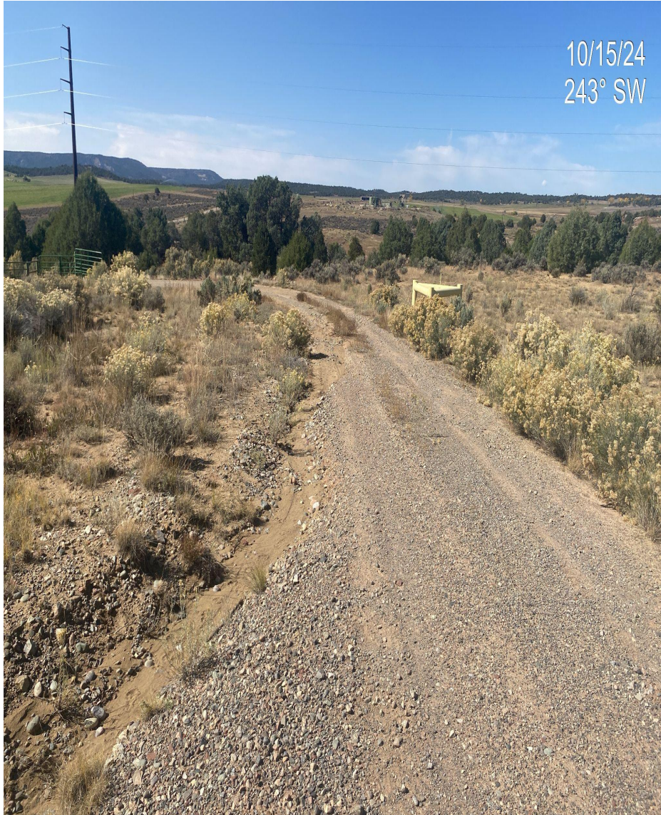
Photo 3. Stormwater issues observed along the access road. Evidence of sediment transport and deposition. Additional stormwater BMPs along the access road are needed.
