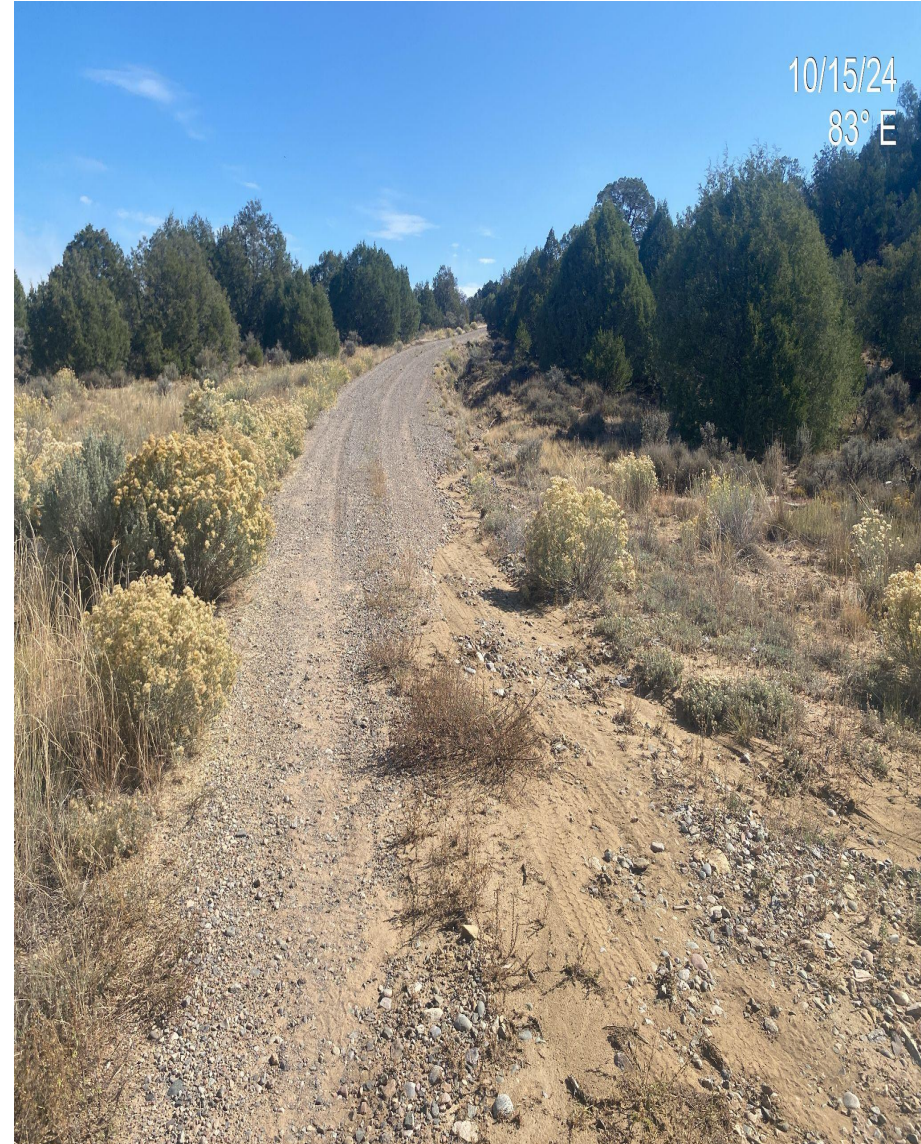
Photo 3. Stormwater issues observed along the access road. Evidence of sediment transport and deposition. Additional stormwater BMPs along the access road are needed.
