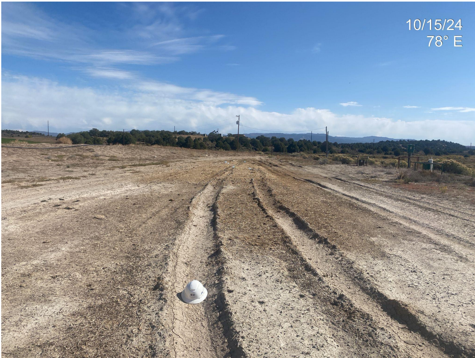
Photo 3. Rutting occurring on the active pad.
