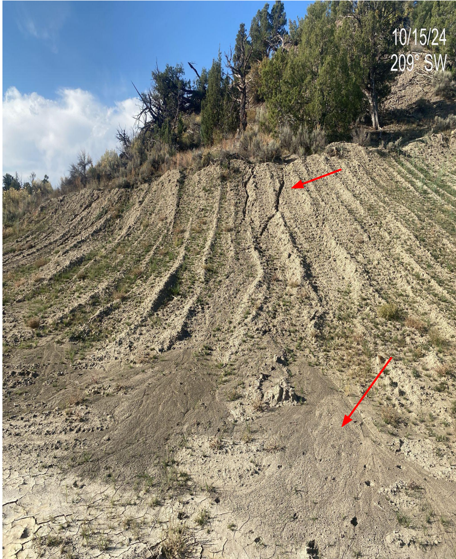
Photo 4. View of rill erosion and sediment transportation observed in the location fill and cut slopes, additional stabilization/stormwater BMPs needed in these areas.
