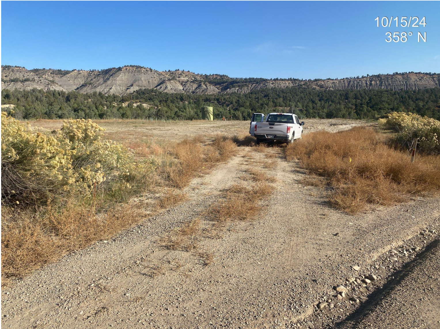
Photo 6. View of access point that has not been reclaimed including gravel removal, recontouring or decompaction. Weedy kochia debris in the southern corner.
