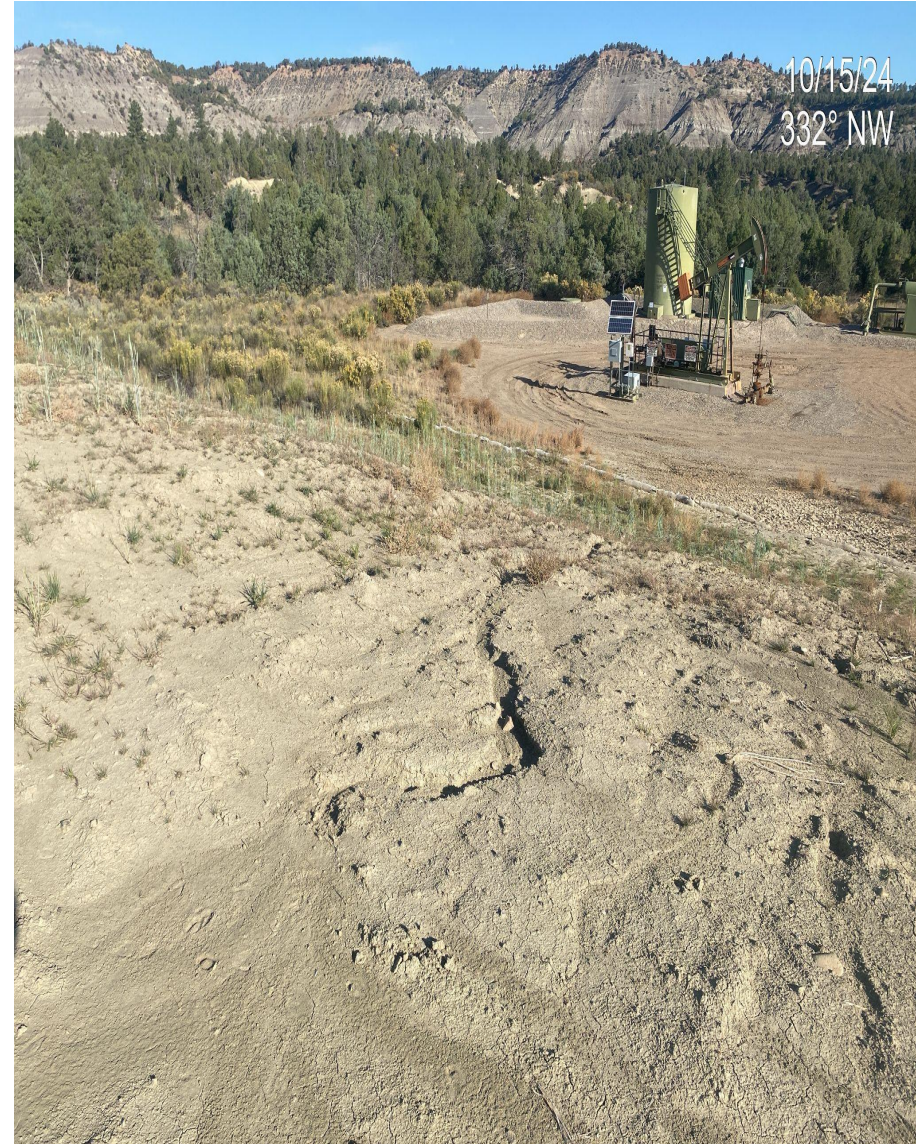
Photo 4. View of rill erosion and sediment transportation observed in the location fill and cut slopes, additional stabilization/stormwater BMPs needed in these areas.
