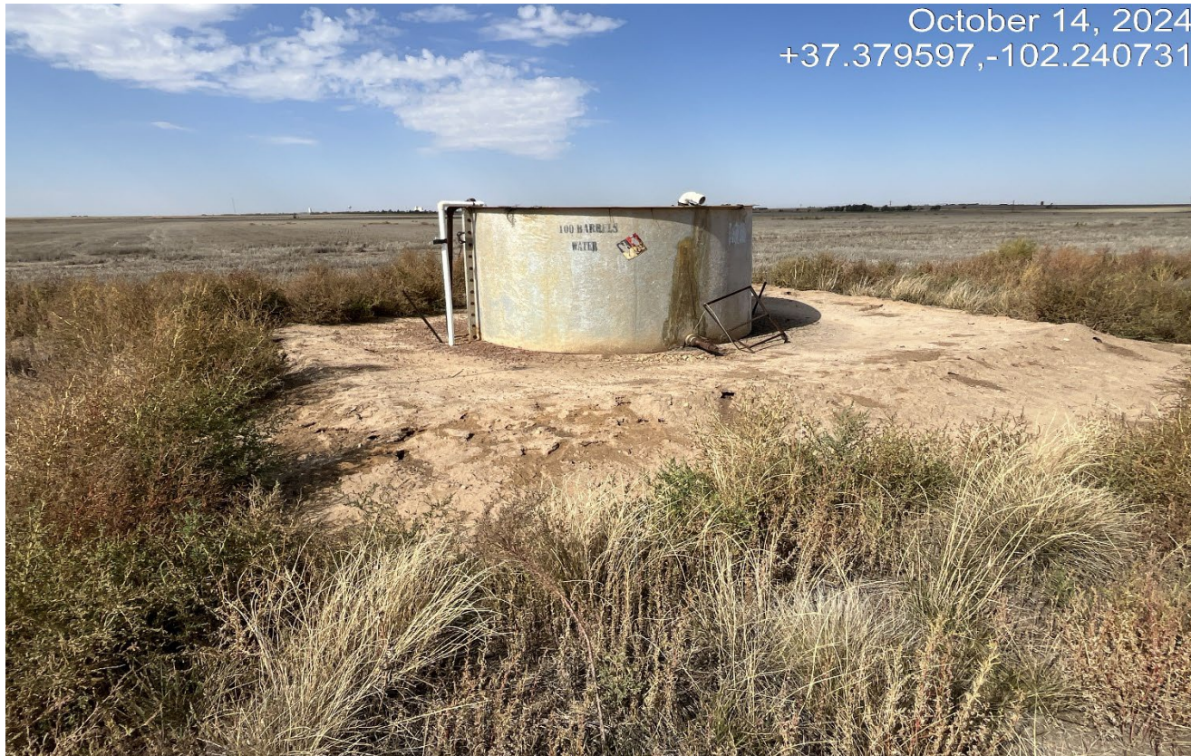
Photo 1. Facing toward the tank battery approx. 1200' east of the wellsite. There is insufficient secondary containment of the tank.
