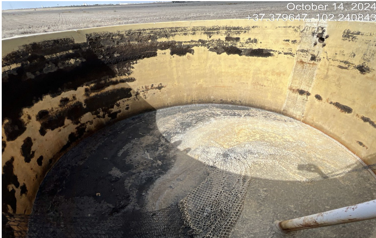
Photo 2. There is no netting on the open top tank contains a hardened E&P substance.
