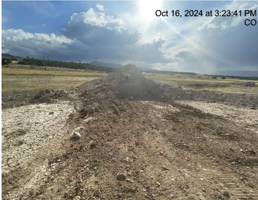
Photo # 6293 Stockpiled soils with no BMP's
