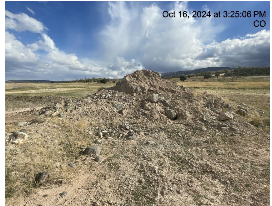
Photo # 6296 Stockpiled soils with no BMP's
