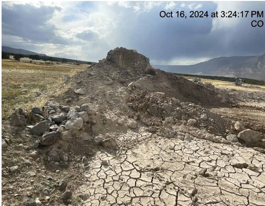
Photo # 6295 Stockpiled soils with no BMP's
