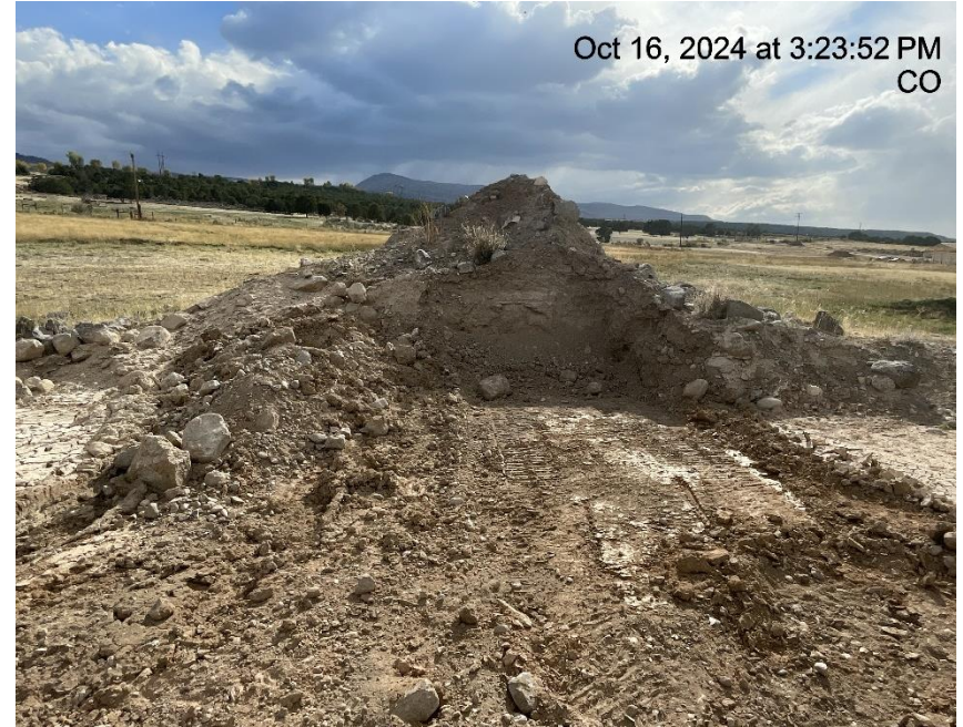
Photo # 6294 Stockpiled soils with no BMP's
