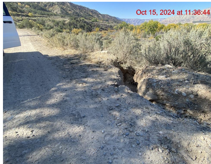
Insufficient Erosion Control – Photo #04234
