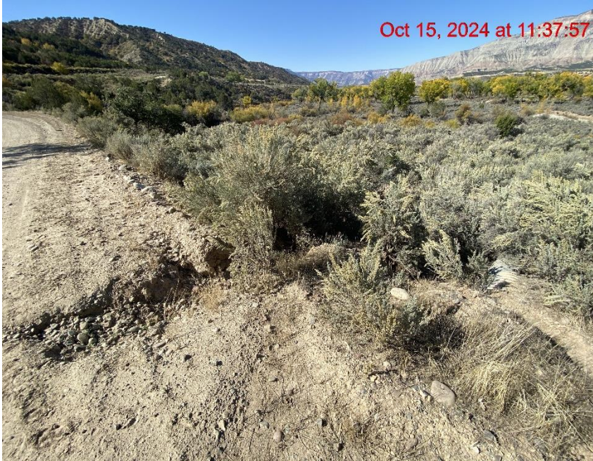
Insufficient Erosion Control/Transport of Sediment from Lease Road – Photo #04238
