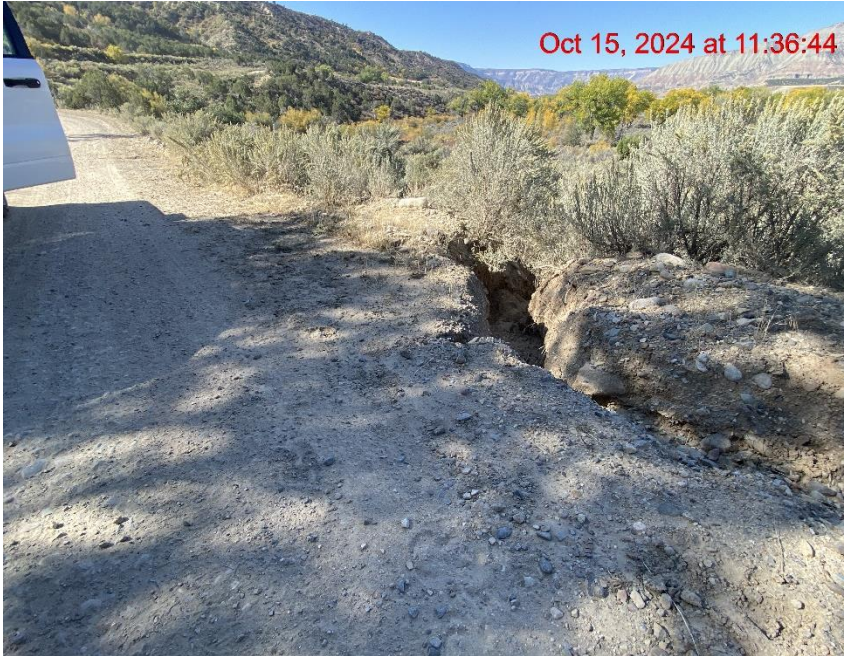
Insufficient Erosion Control – Photo #04234
