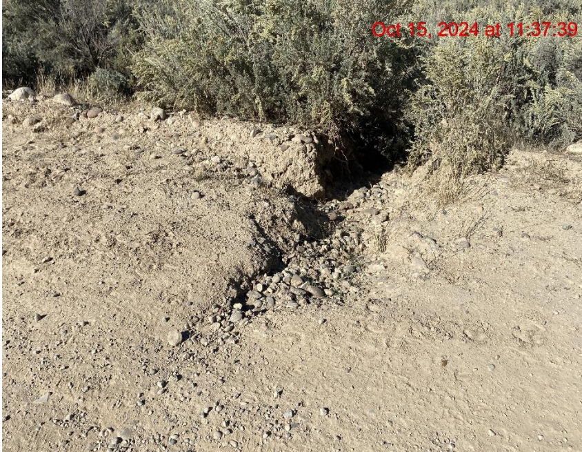
Insufficient Erosion Control/Transport of Sediment from Lease Road – Photo #04237
