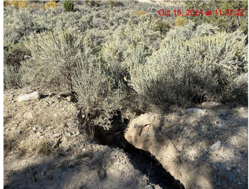
Insufficient Erosion Control/Transport of Sediment from Lease Road – Photo #04236
