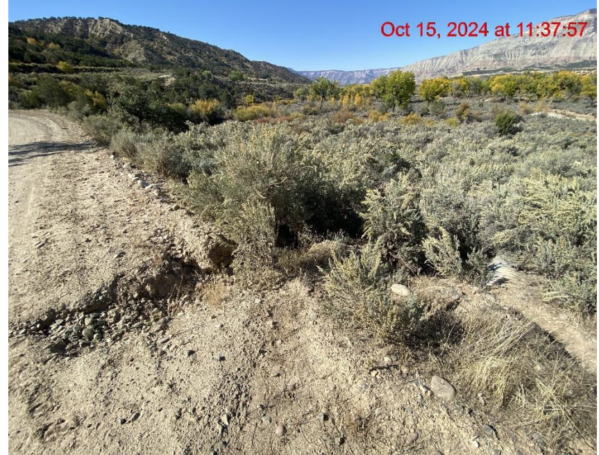
Insufficient Erosion Control/Transport of Sediment from Lease Road – Photo #04238
