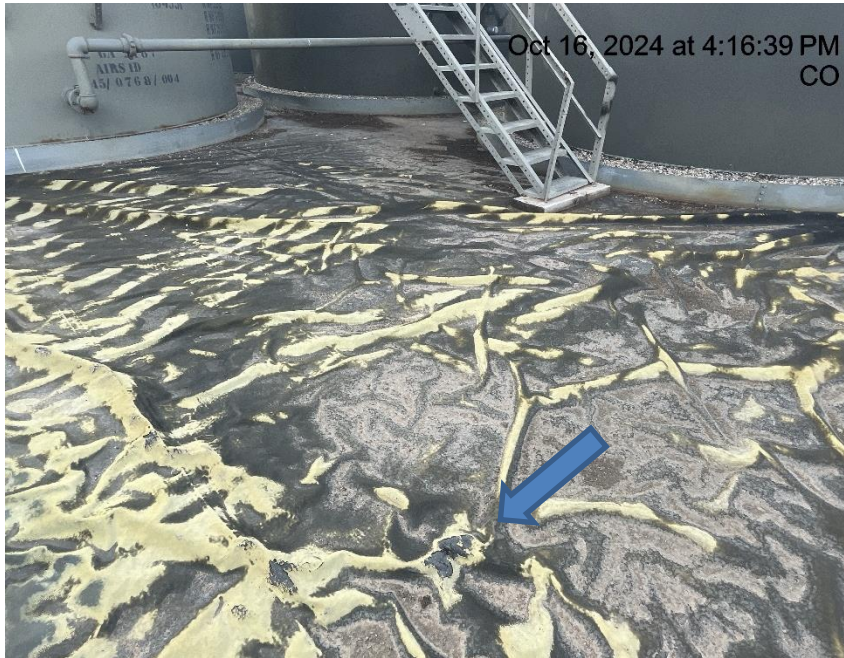
Photo # 6502 Hole in liner/liner needs maintenance
