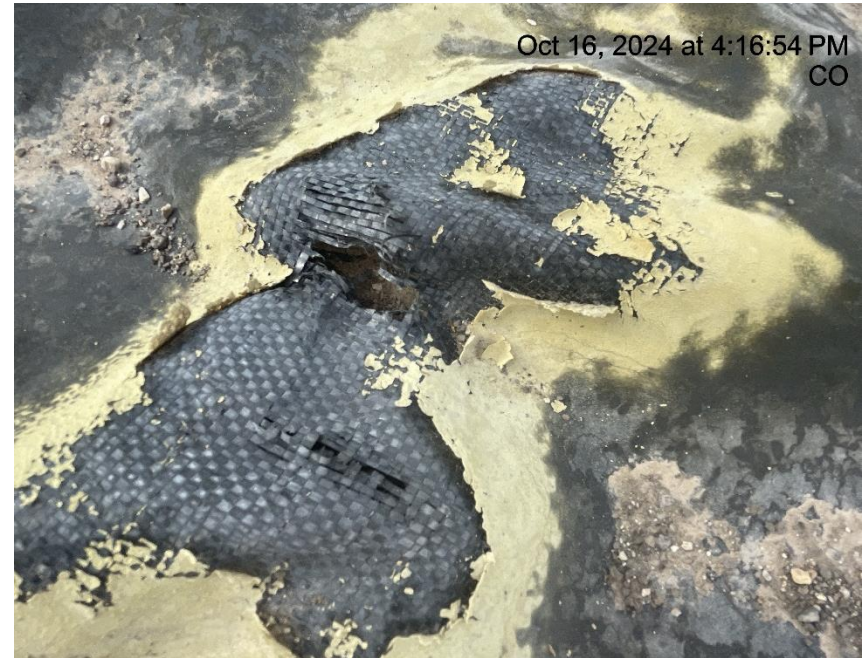
Photo # 6503 Hole in liner/liner needs maintenance
