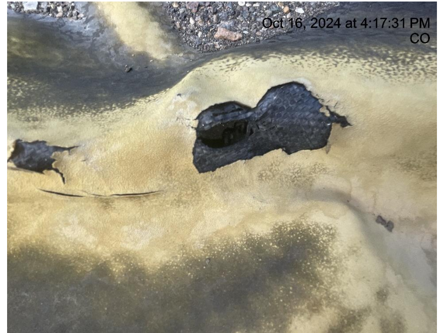
Photo # 6505 Hole in liner/liner needs maintenance
