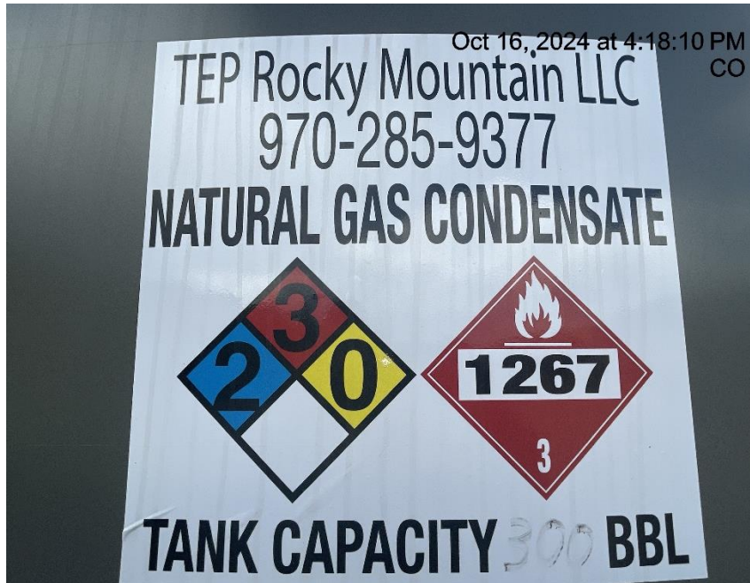
Photo # 6506 Capacity on tank label fading & becoming illegible
