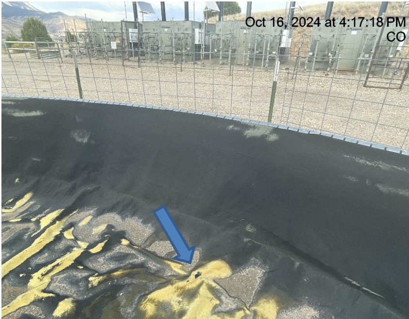
Photo # 6504 Hole in liner/liner needs maintenance
