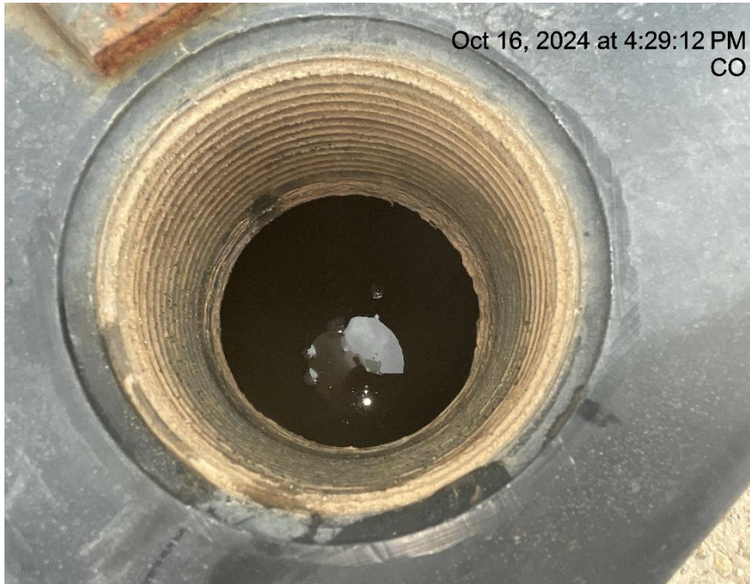
Photo # 6507 Failure to maintain chemical BMP - Chemical tank containment approximately 3/4 th full of fluid/BMP insufficient to contain possible spill
