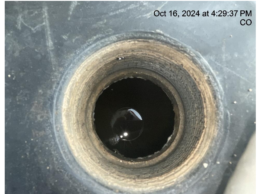
Photo # 6508 Failure to maintain chemical BMP - Chemical tank containment approximately 3/4 th full of fluid/BMP insufficient to contain possible spill
