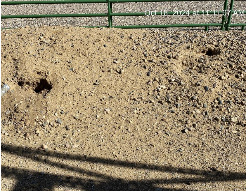
Burrows in tank berm
