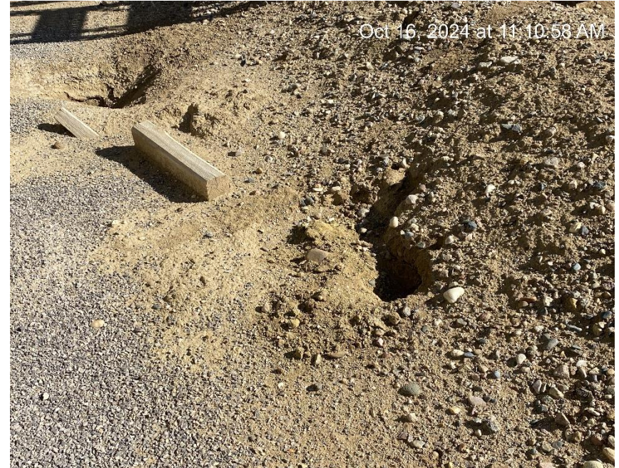
Burrows inside tank berm
