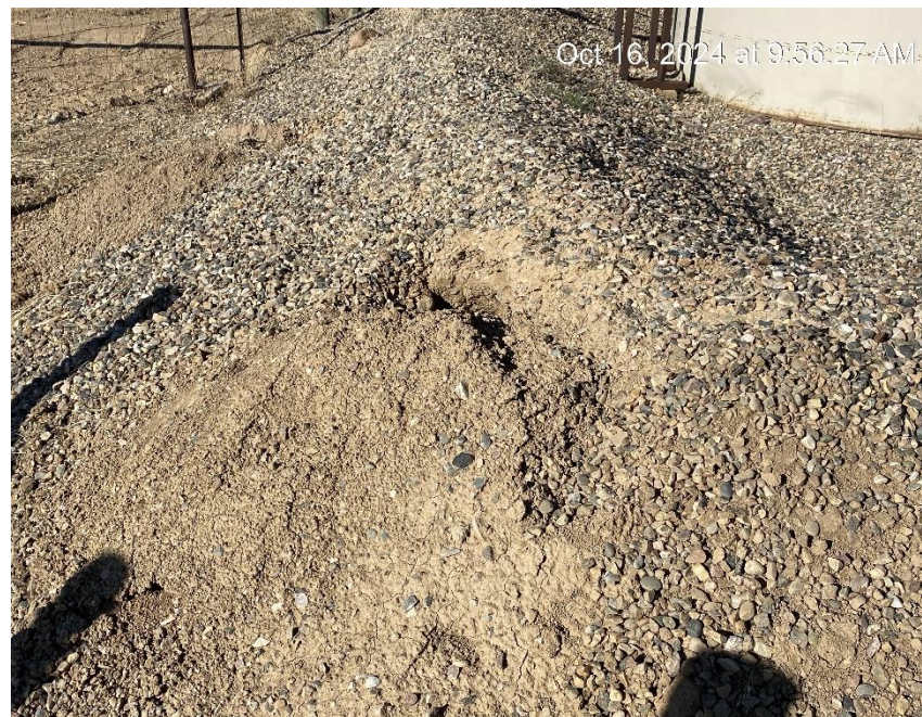
Rodent burrows in tank berm
