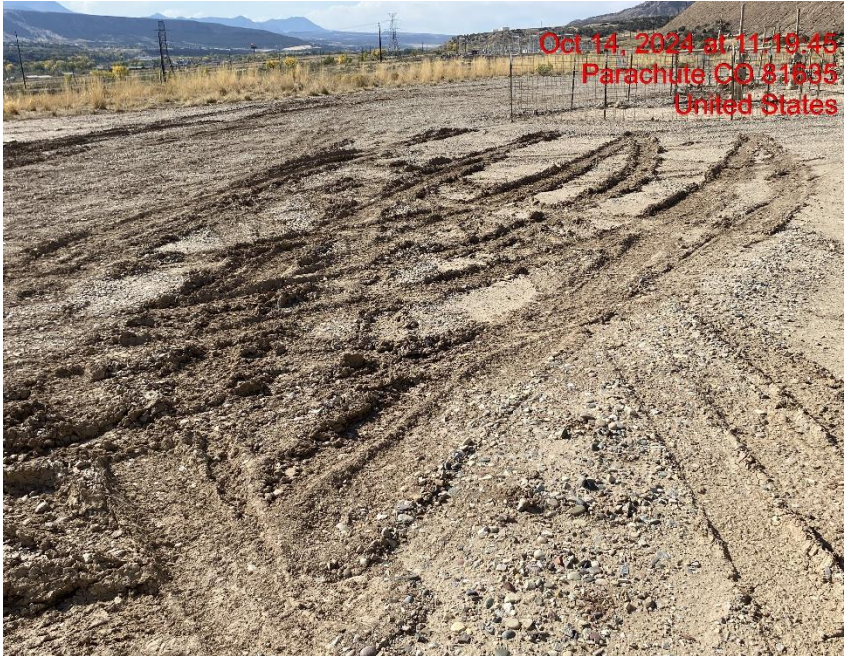
Lack of Stabilization – Photo #04178
