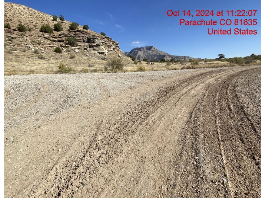
Insufficient Tracking BMPs – Photo #04183
