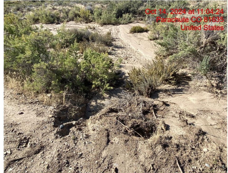
Insufficient Erosion Control/Transport of Sediment From Lease Road – Photo #04166
