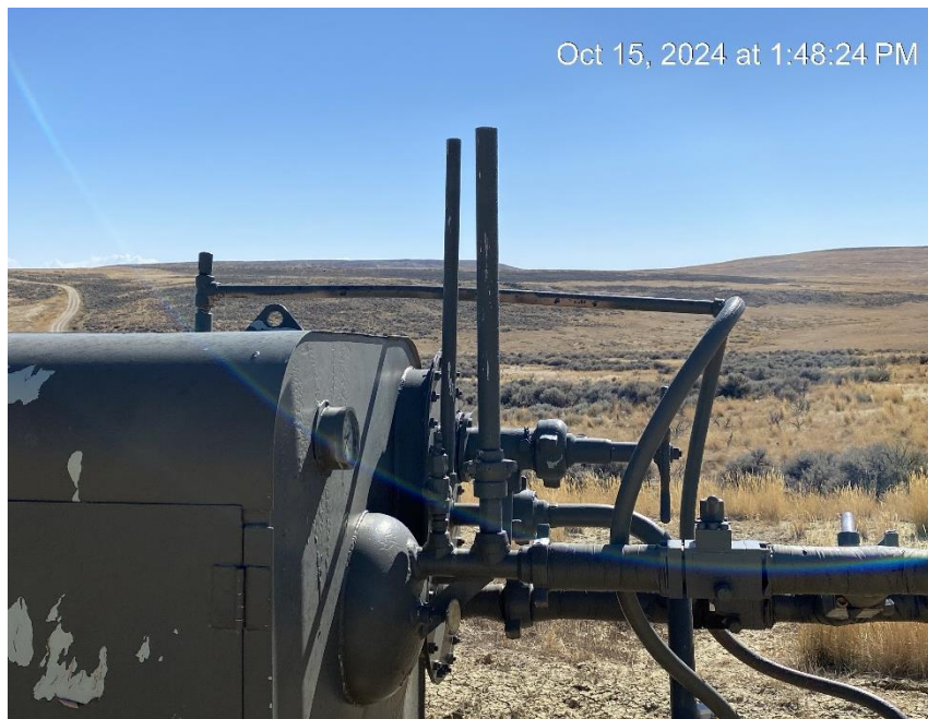
Risers missing rain caps
