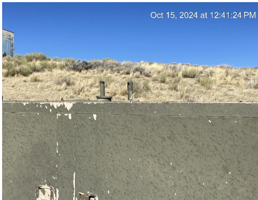
Vent riser missing cap
