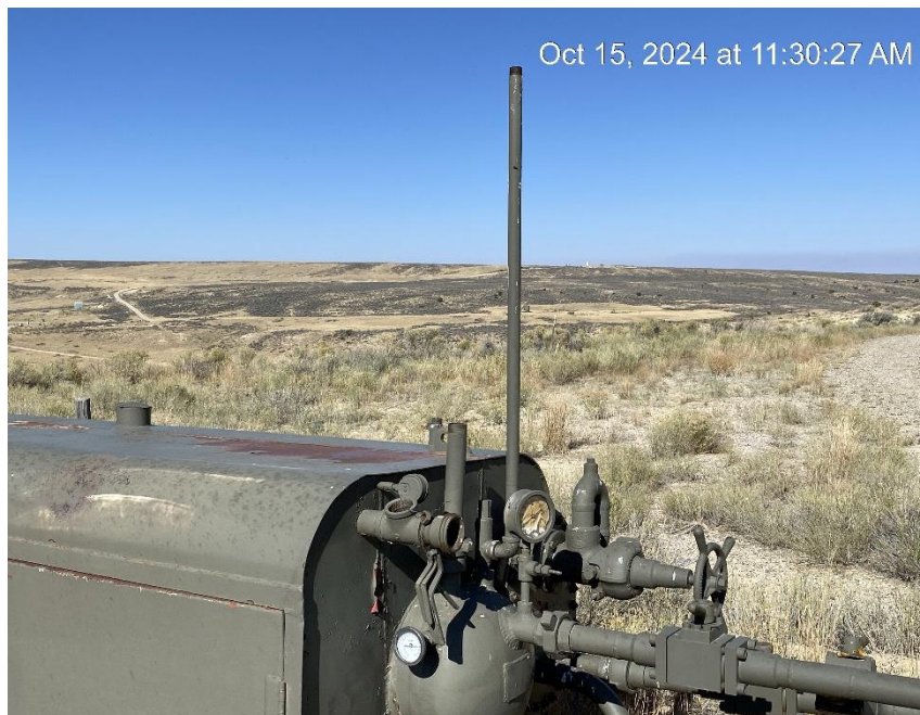
Relief vent risers missing protective caps
