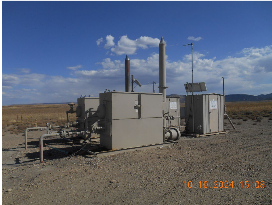
Separators and Meter housings
