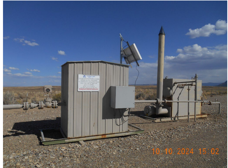
Separator and Meter housing
